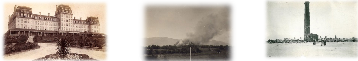
Figure 6 - Raymond Hotel - Before, During, and After Fire
