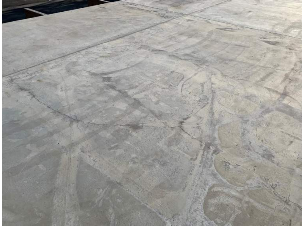
(Gar-5) Roof of Reservoir
