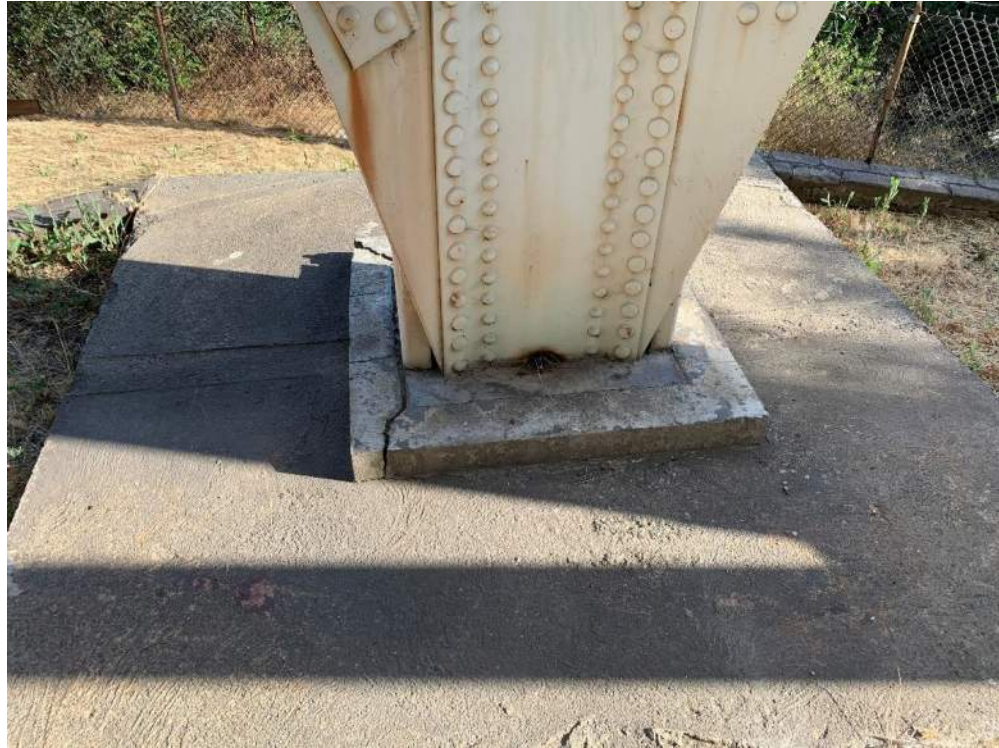
(Ray-9) Base of Column of Elevated Tank
