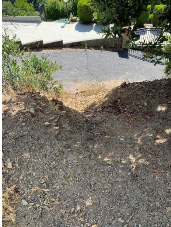
(Bil-3) Access Road from Top of Tank Site
