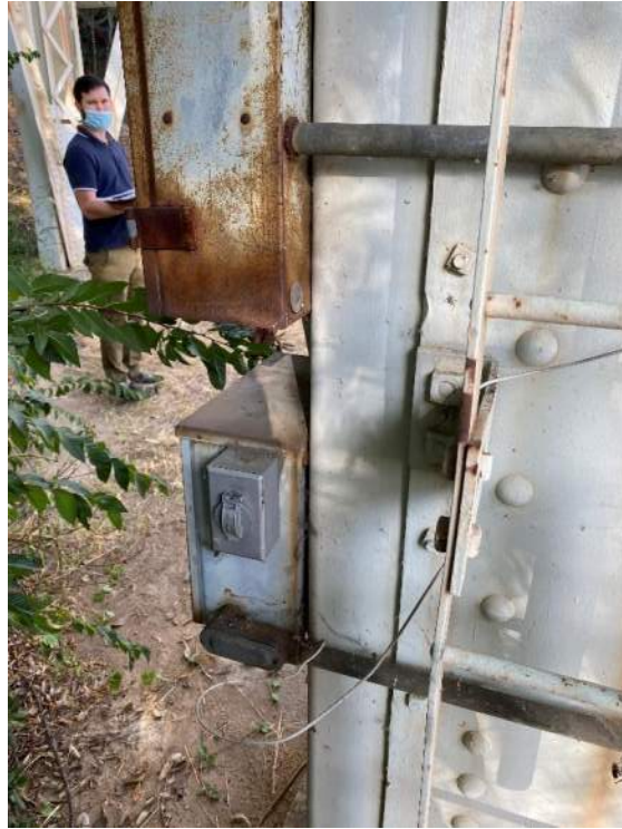
(Ray-21) Access Ladder to Elevated Tank
