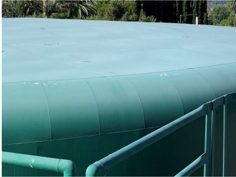
(Grand-3) Top of Reservoir 2
