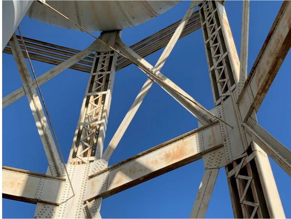
(Ray-1) Elevated Tank
