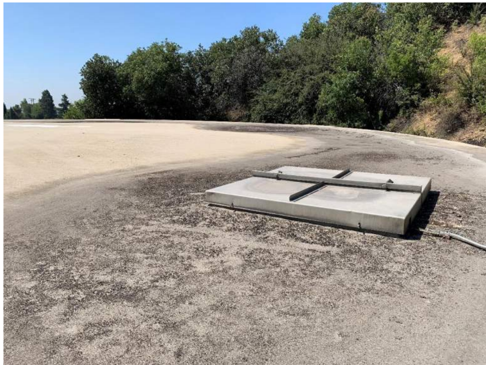
(West-2) Access Hatch on top of Reservoir
