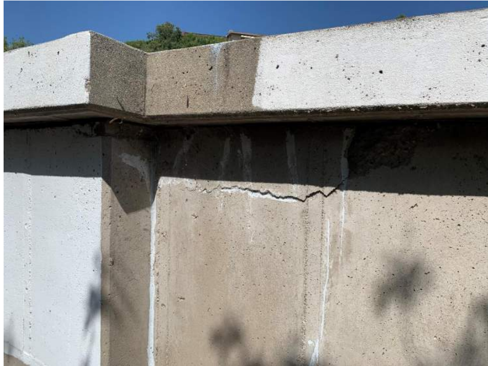
(West-9) Top Wall of Reservoir
