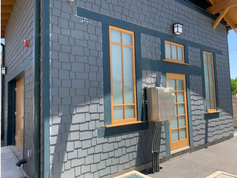
(Wil-3) Exterior of Pump Room
