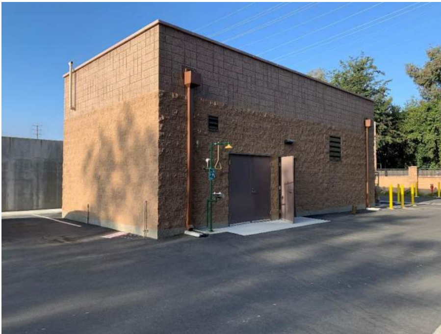
(Gar-8) Outside of Chemical/Pump Room
