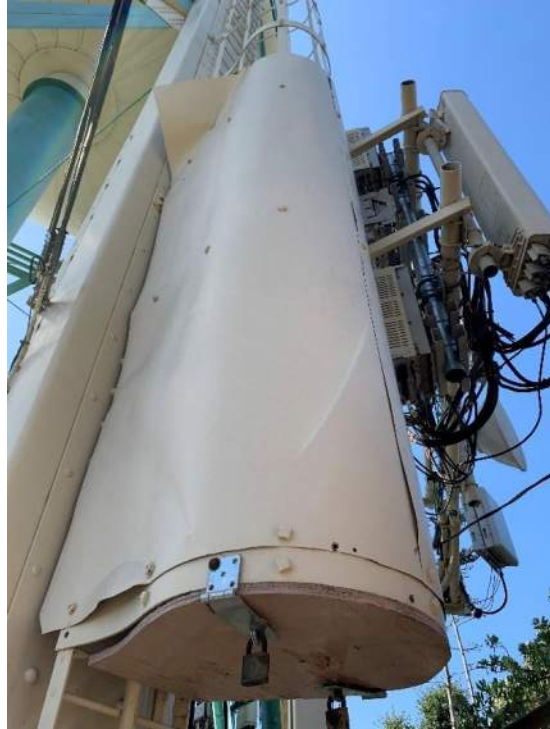
(Bil-7) Access Ladder to Tank and Antenna
