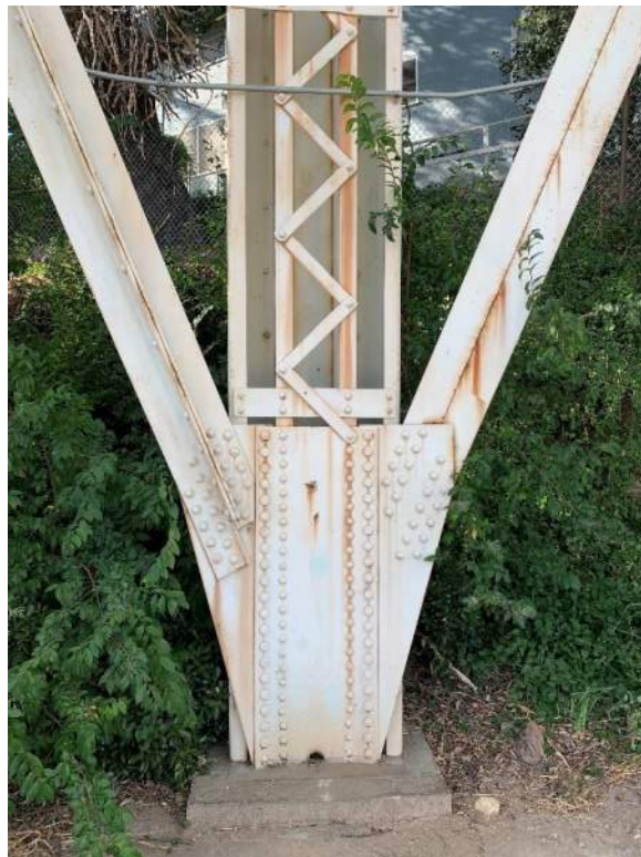
(Ray-6) Column of Elevated Tank
