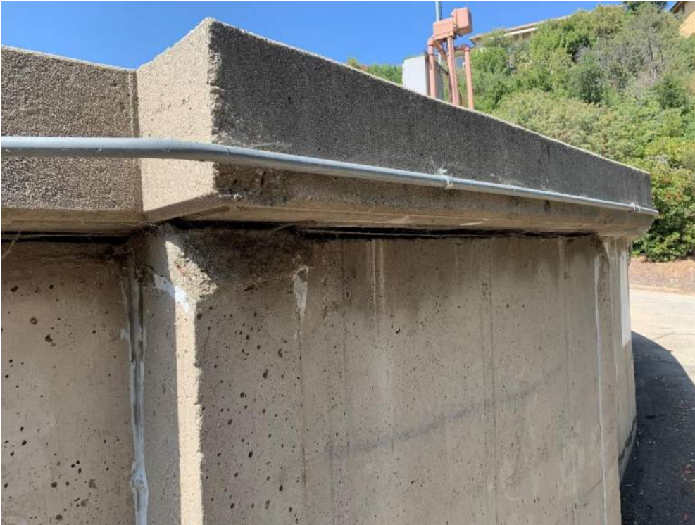
(West-7) Top Wall of Reservoir
