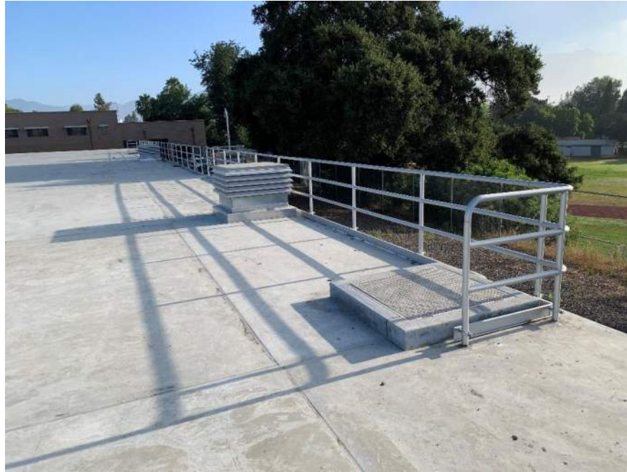
(Gar-9) Access Hatch on Reservoir Roof
