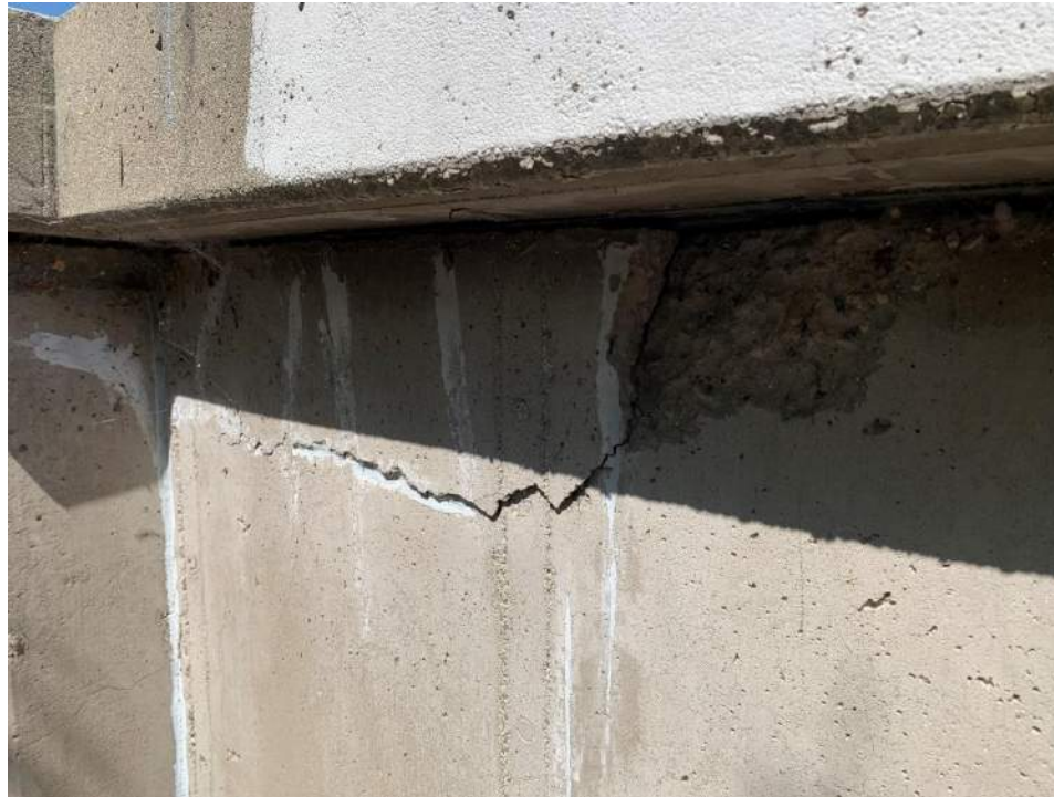
(West-10) Top Wall of Reservoir
