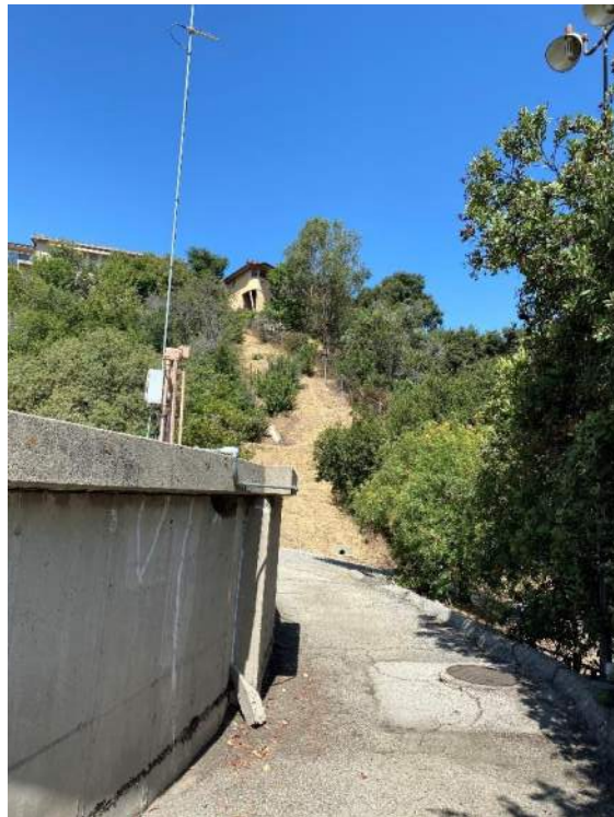
(West-18) Antenna on top of Reservoir
