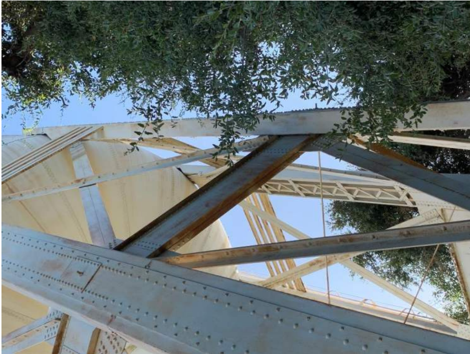
(Ray-3 ) Elevated Tank
