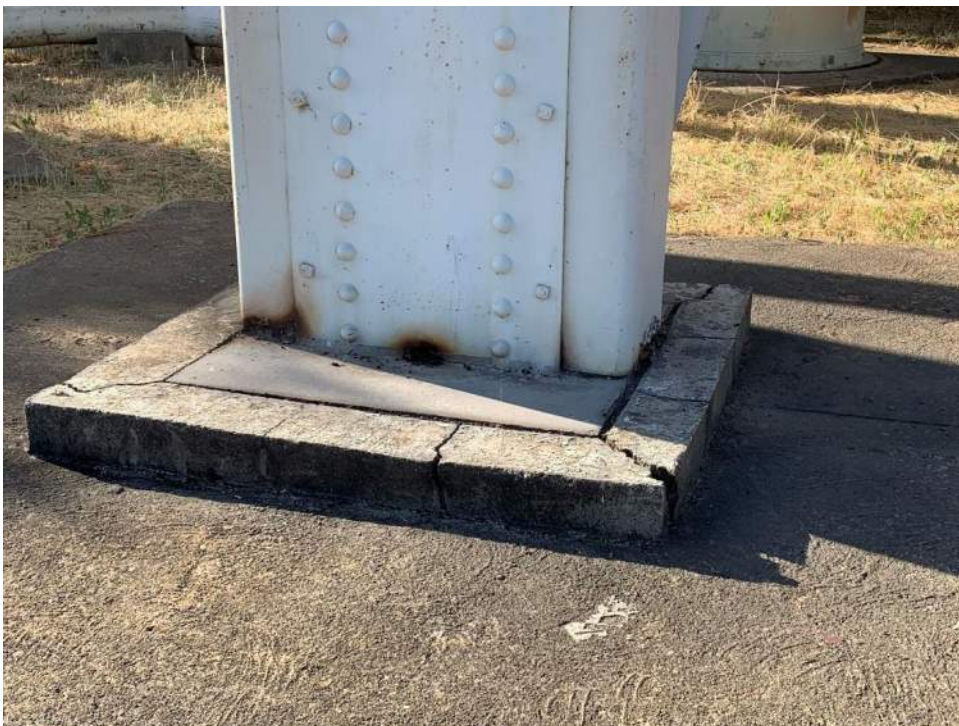
(Ray-4) Base of Column of Elevated Tank
