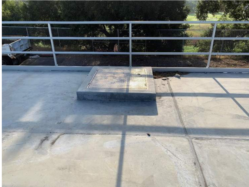
(Gar-1) Access Hatch on top of Reservoir.
