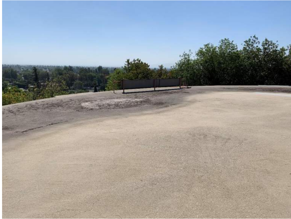
(West-5) Roof of Reservoir
