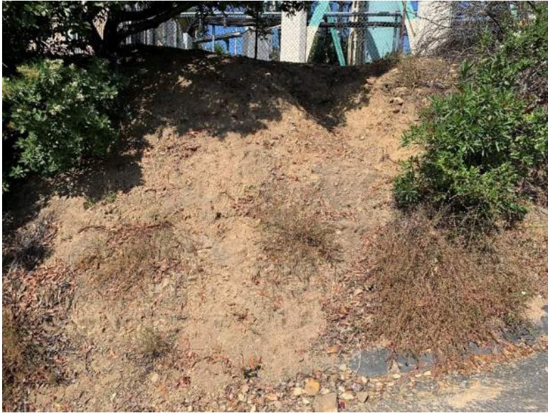
(Bil-1) Edge of Slope Below Tank Site
