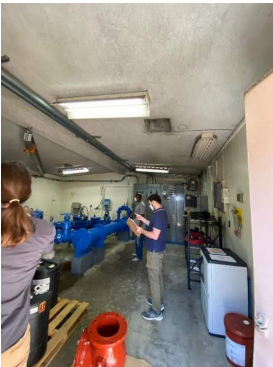
(West-24) Inside of Pump Room
