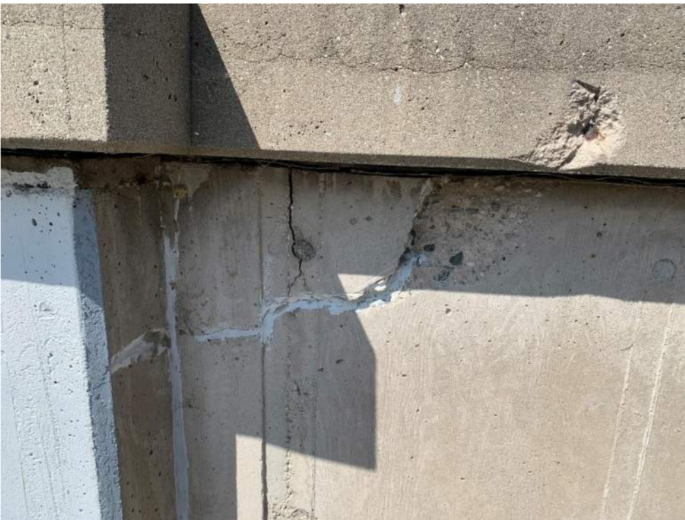
(West-8) Top Wall of Reservoir
