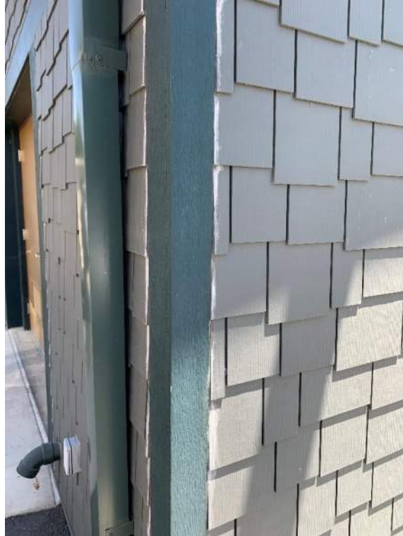
(Wil-1) Exterior of Pump Room
