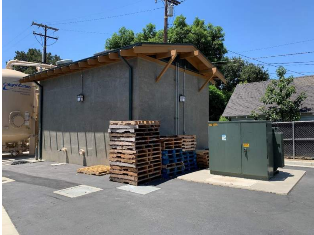
(Wil-5) Electrical Supply and Storage Room
