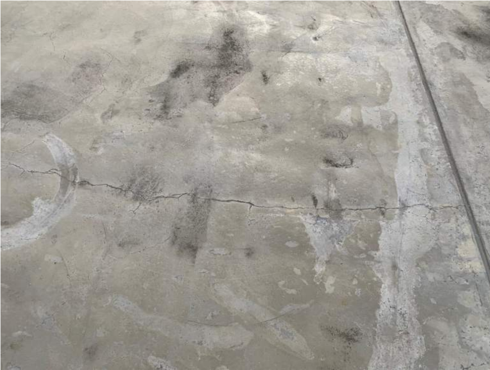
(Gar-3) Roof of Reservoir
