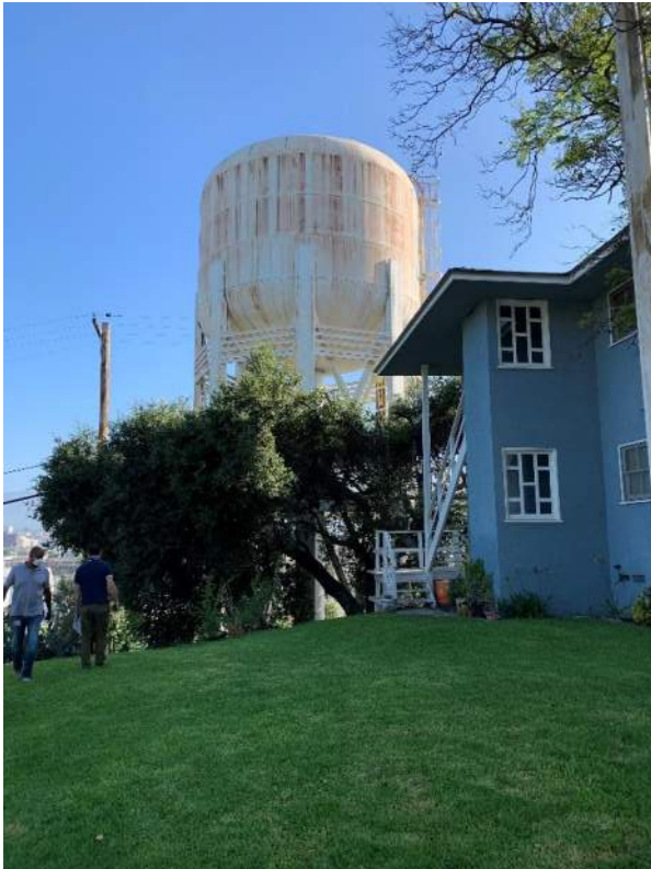
(Ray-11) Elevated Tank – From Roadway
