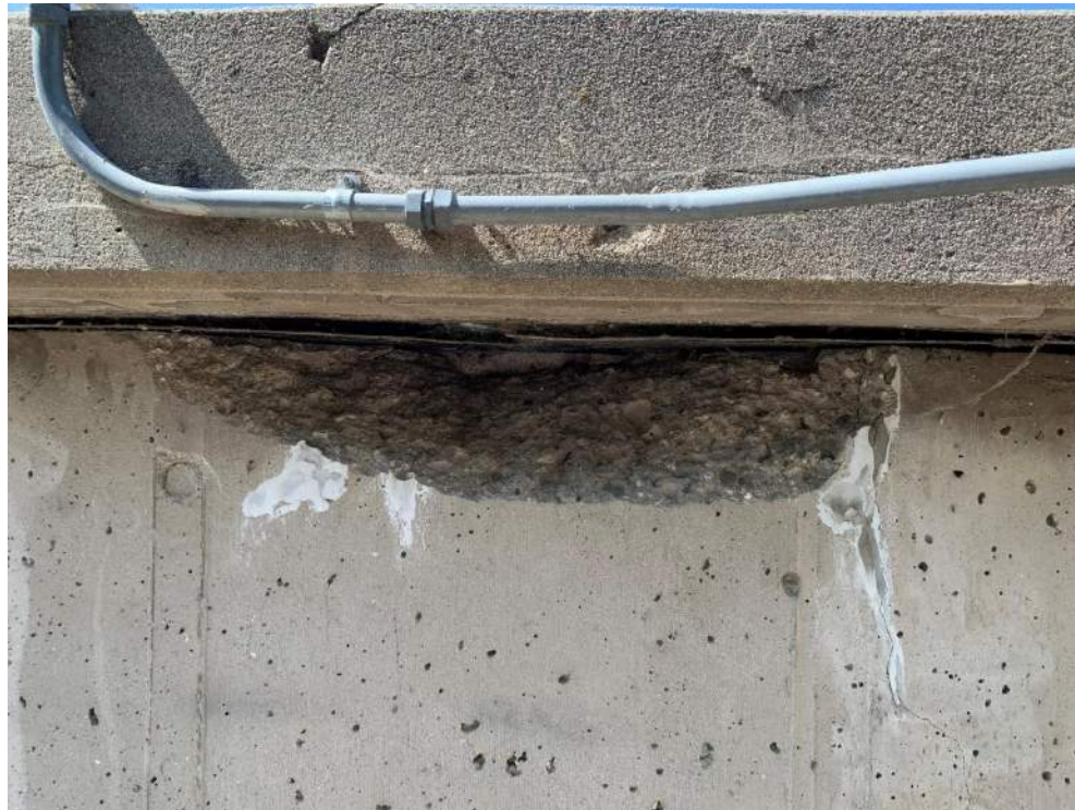
(West-6) Top Wall of Reservoir
