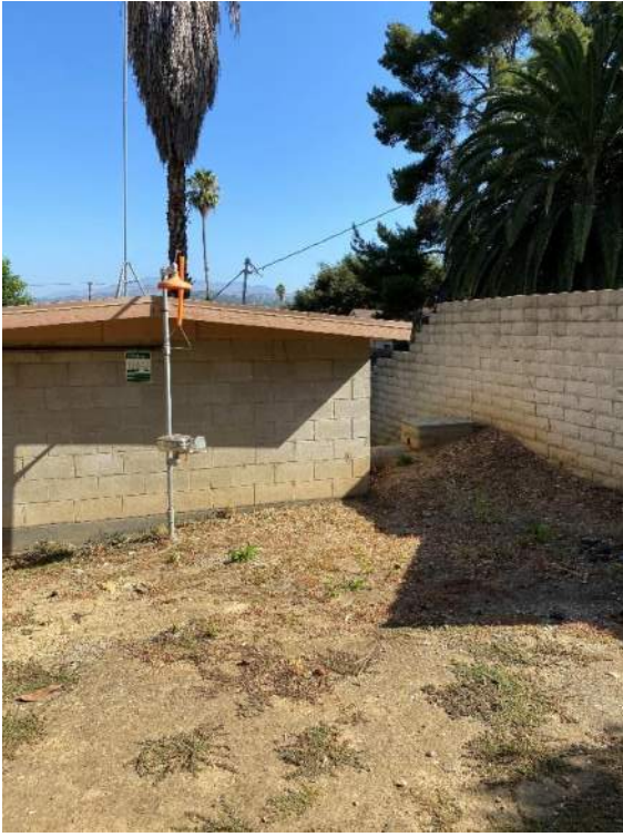
(Kol-9) Side View of Metering Building
