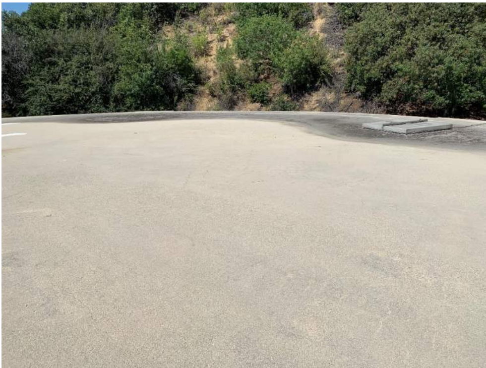
(West-4) Roof of Reservoir
