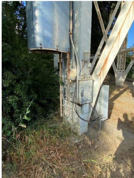
(Ray-18) Access Ladder to Elevated Tank
