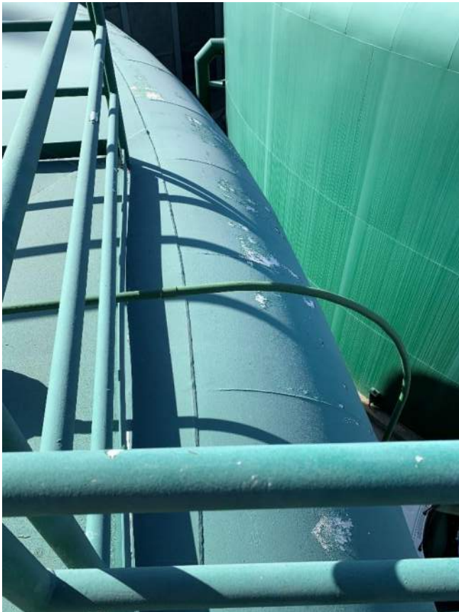
(Grand-2) Top of Reservoir 1
