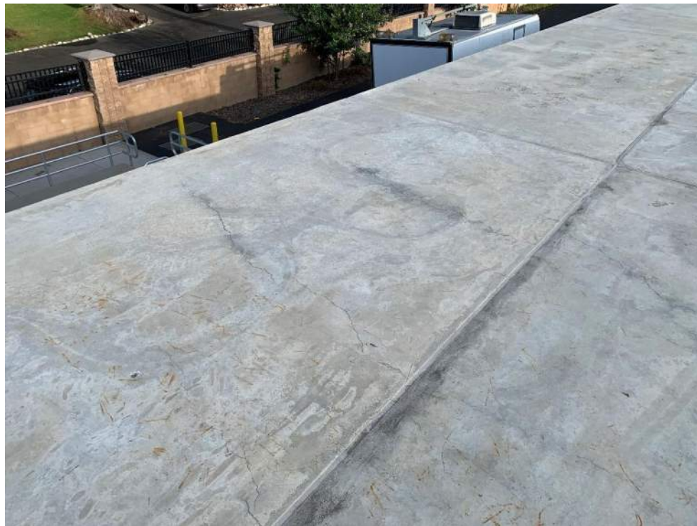
(Gar-6) Roof of Reservoir
