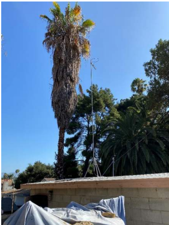
(Kol-22) Antenna on top of Metering Building
