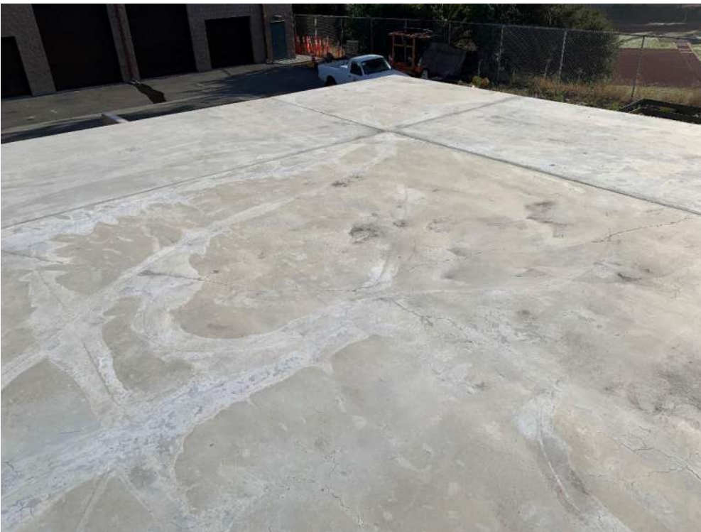
(Gar-4) Roof of Reservoir
