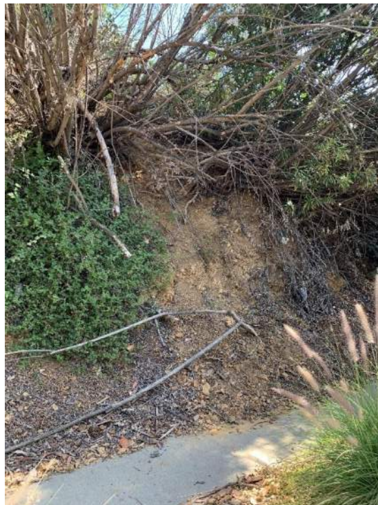
(Bil-4) Slope Around Tank Site
