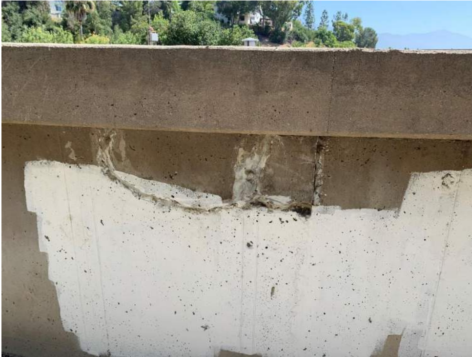
(West-11) Top Wall of Reservoir
