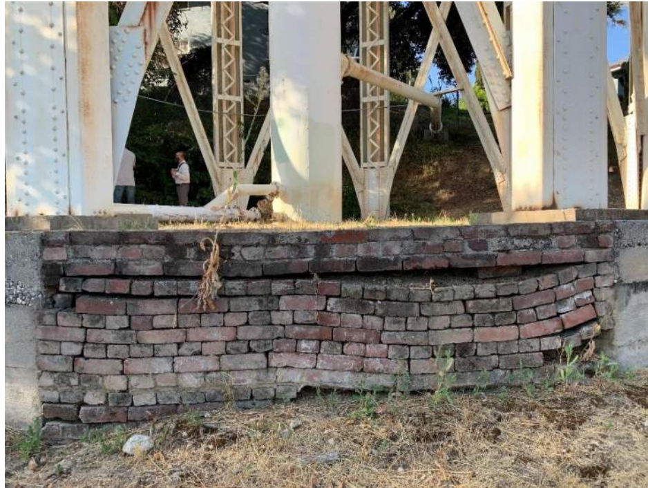
(Ray-5) Retaining Wall at Base of Elevated Tank
