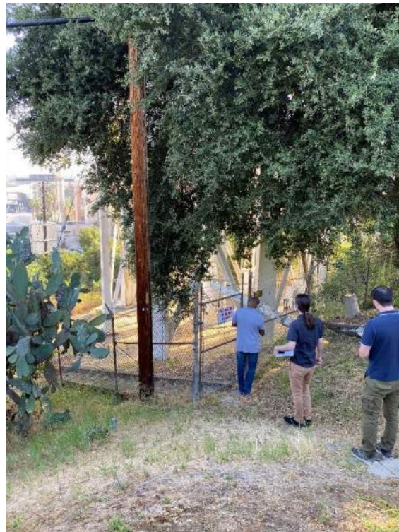
(Ray-22) Outside of Tank Site
