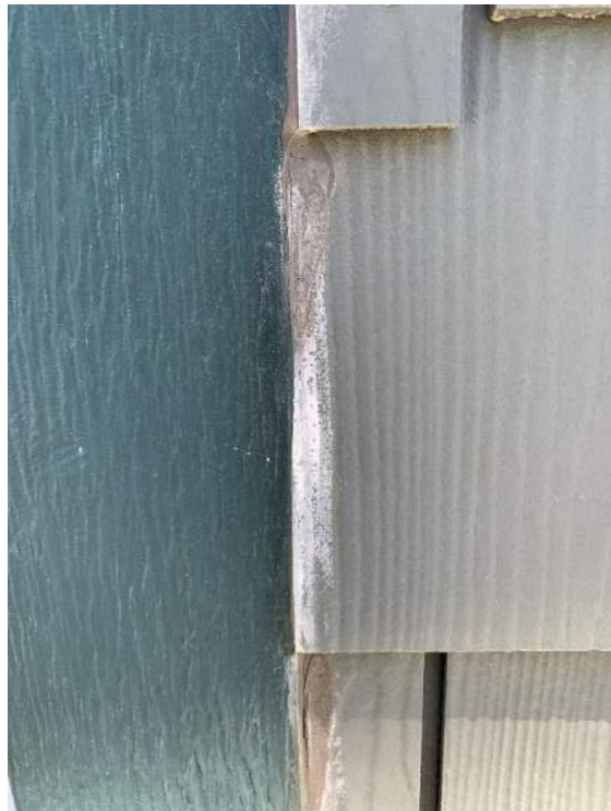
(Wil-2) Exterior of Pump Room
