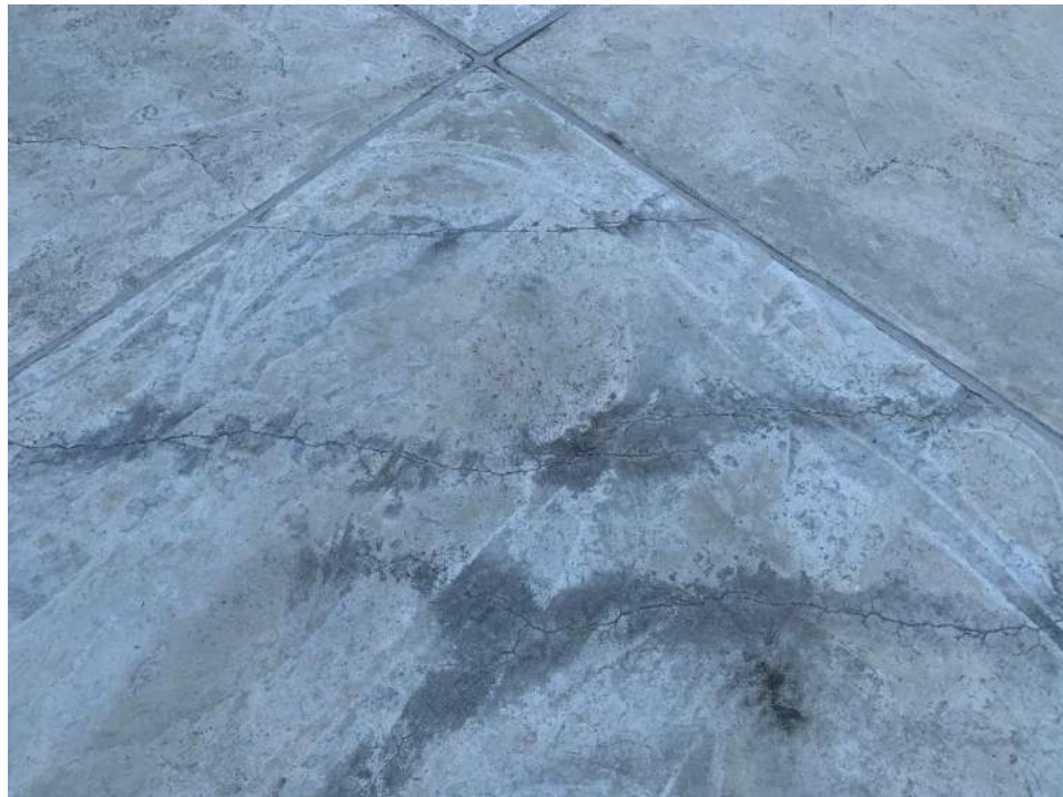
(Gar-2) Roof of Reservoir
