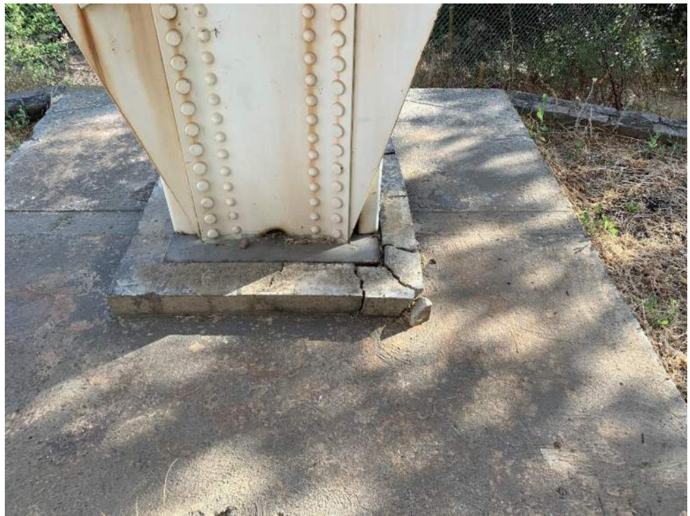
(Ray-10) Base of Column of Elevated Tank
