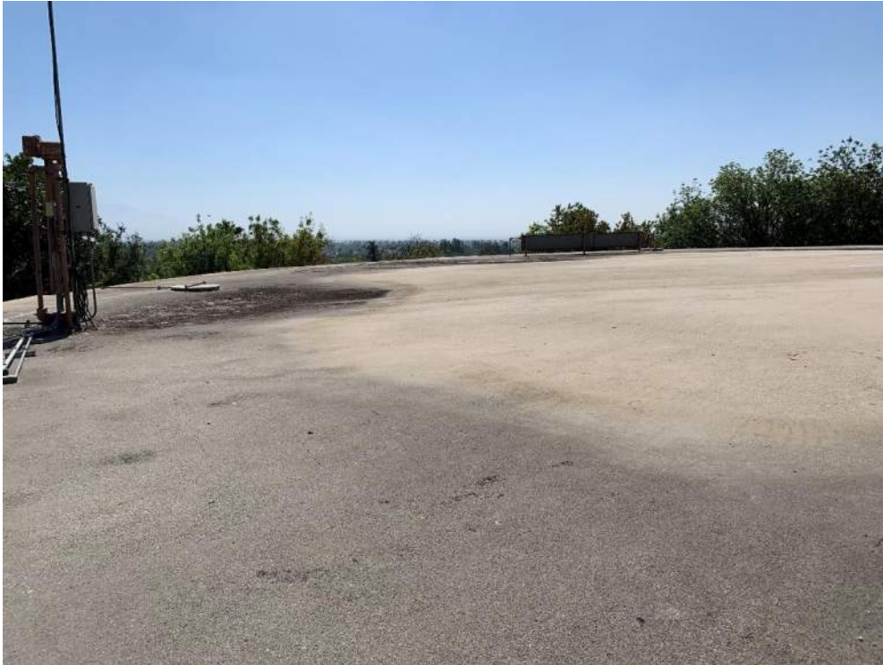
(West-3) Roof of Reservoir
