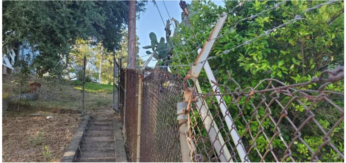
(Ray-13) Stairway Access to Tank
