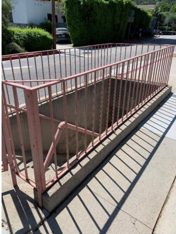
(Ind-3) Site Access Stairway
