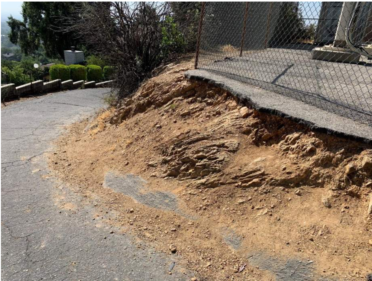
(Bil-2) Driveway and Slope Below Tank Site
