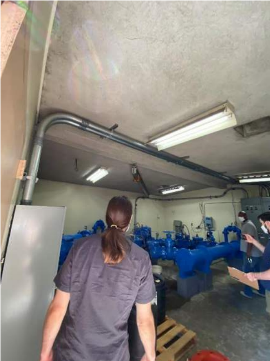
(West-19) Inside of Pump Room
