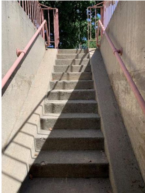
(Ind-4) Site Access Stairway
