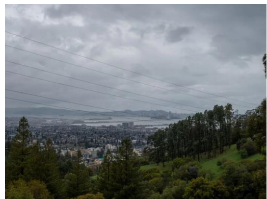
Figure 4: Powerlines cross the hills along Grizzly Peak Boulevard. Credit: Ximena Natera, Berkeleyside/CatchLight
