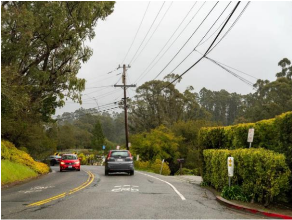
Figure 3: A section of Grizzly Peak Boulevard in the Berkeley Hills that's set to have its utility lines undergrounded. Credit: Ximena Natera. Berkeleyside/CatchLiaht
