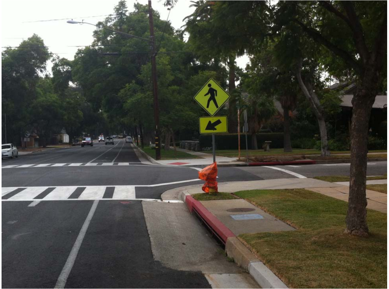
Marengo Ave. looking north
