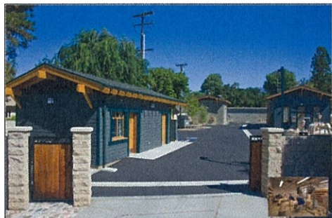
Wilson Reservoir & Pump Station – Complete in 2015
