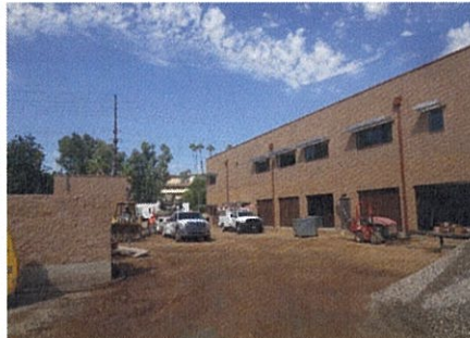
Garfield Reservoir – Under Construction (expected completion October 2017)
