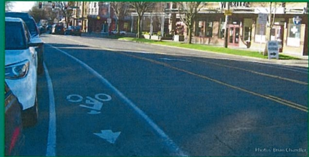
The Stone Way Road Diet improved pedestrian and bicycle safety by incorporating pedestrian refuge islands and a combination of shared lanes and bicycle lanes.
