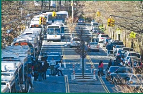
A Road Diet was installed along Luten Avenue to enhance safety for all road users.
