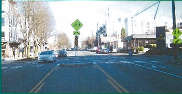
The Stone Way Road Diet improved pedestrian and bicycle safety by incorporating pedestrian refuge islands and a combination of shared lanes and bicycle lanes.
