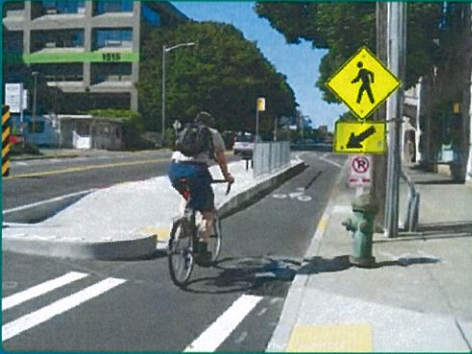
Bicycle lane and floating bus stop
