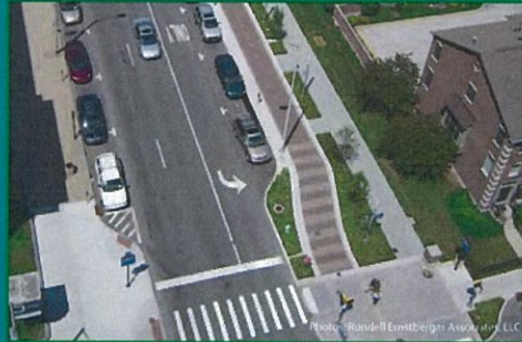
Pedestrian travel is separated from bicycle travel on this segment of ICT.
