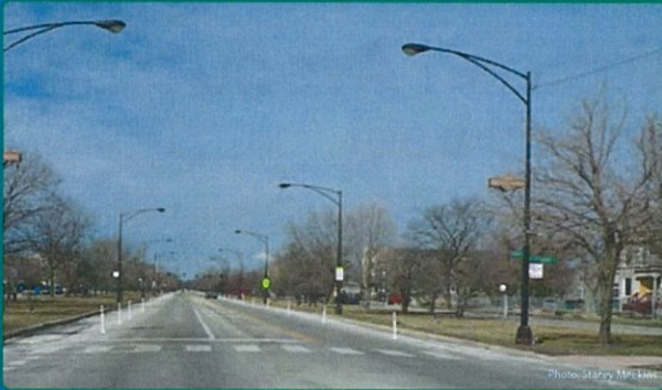
3-lane cross-section with bollard-separated bicycle lanes
