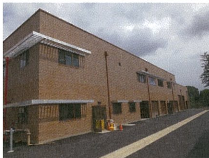
Garfield Reservoir – Under Construction (expected completion November 2017)
