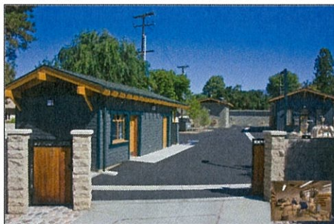
Wilson Reservoir & Pump Station – Complete in 2015
