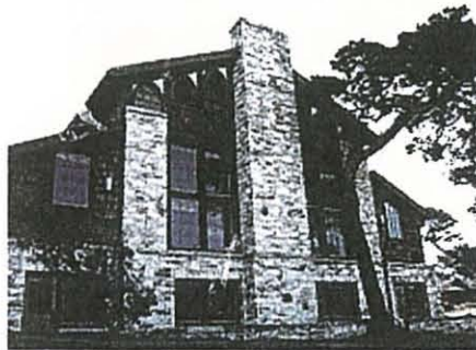
Merrill Hall (1928) on the grounds of Asilomar Conference Center in Pacific Grove, California
