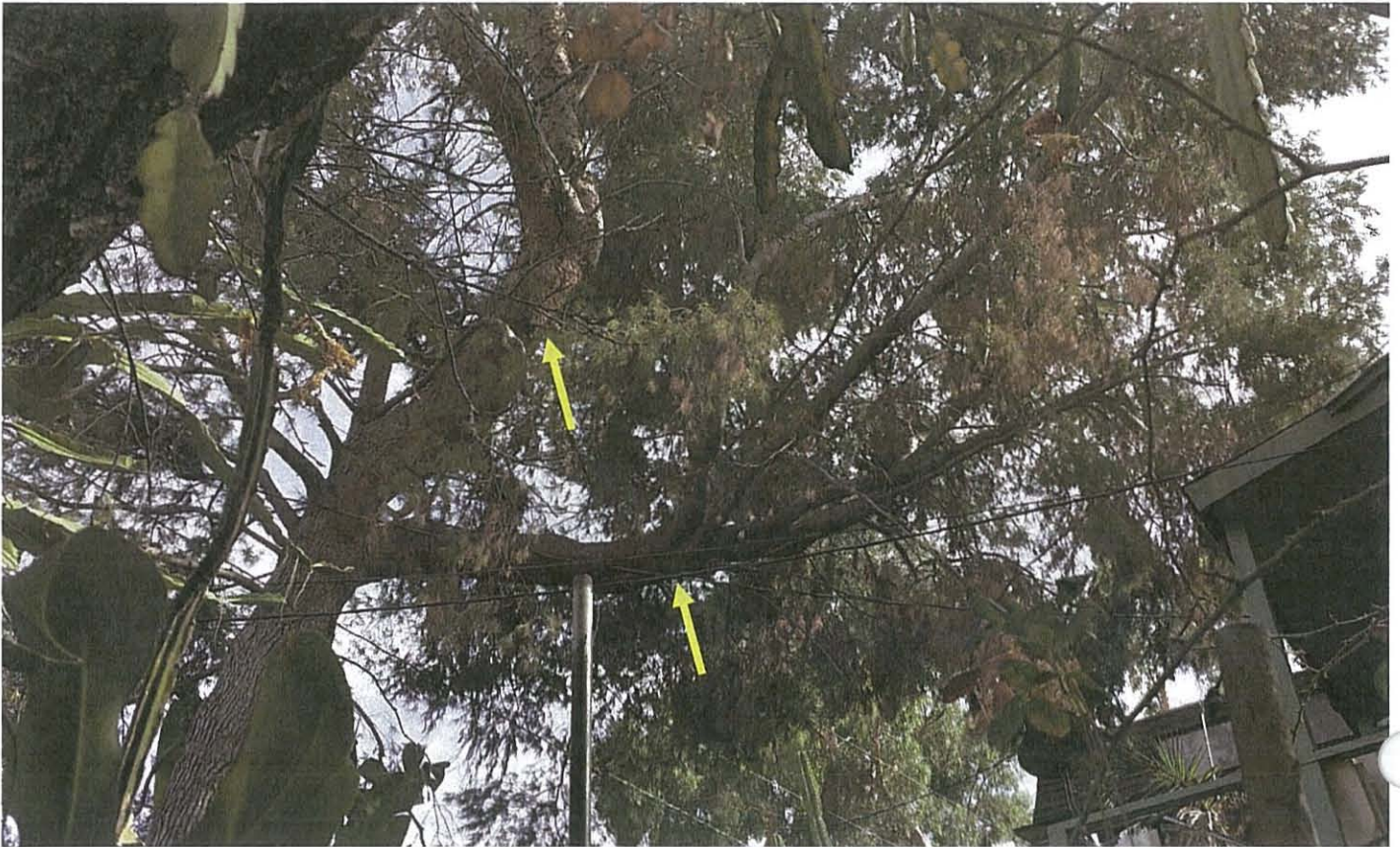
Aleppo pine #32 has 2 codominant trunks which bend heavily west toward the existing structure.
