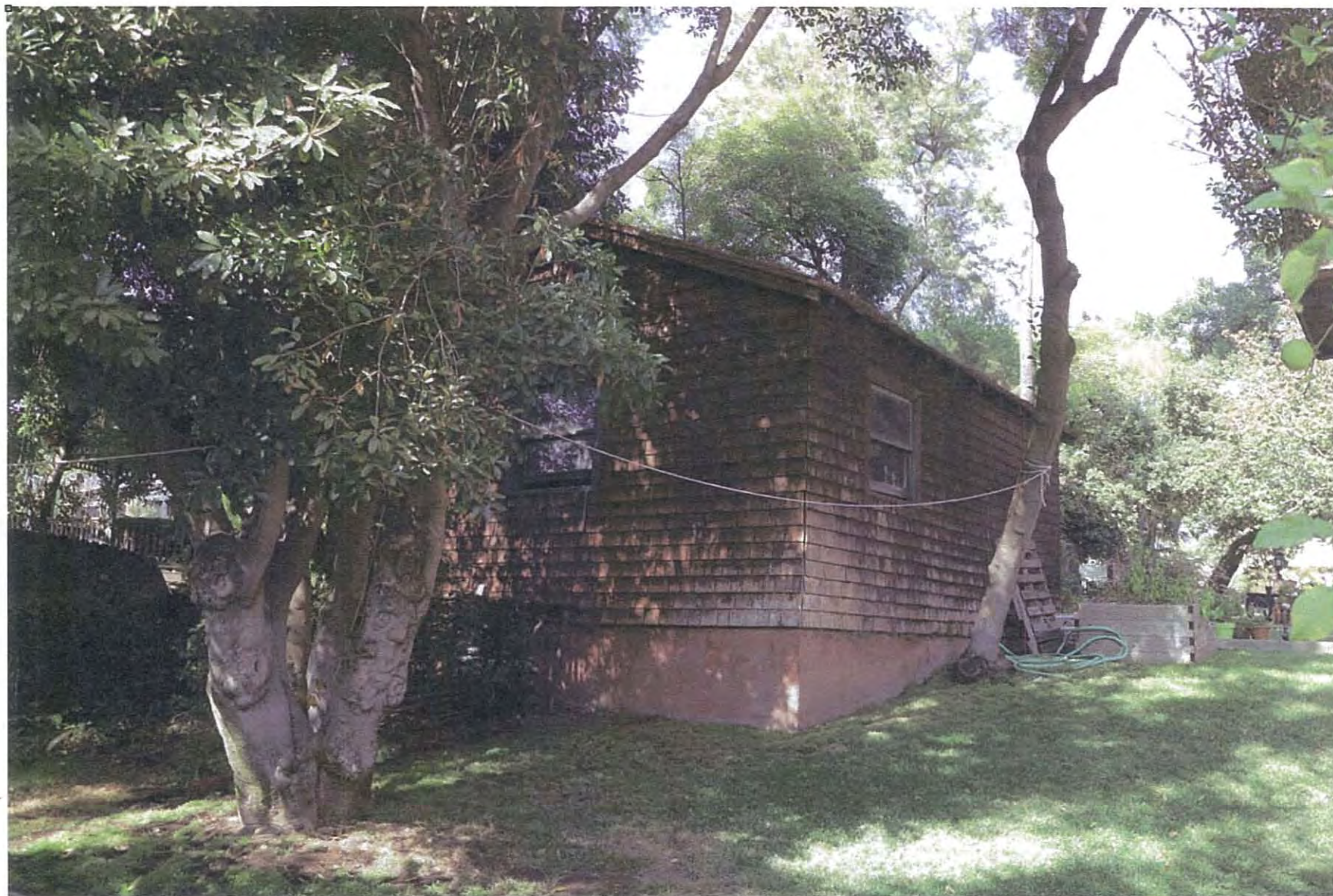
Figure 45 Rear elevation, garage. Northwest portion of parcel.
