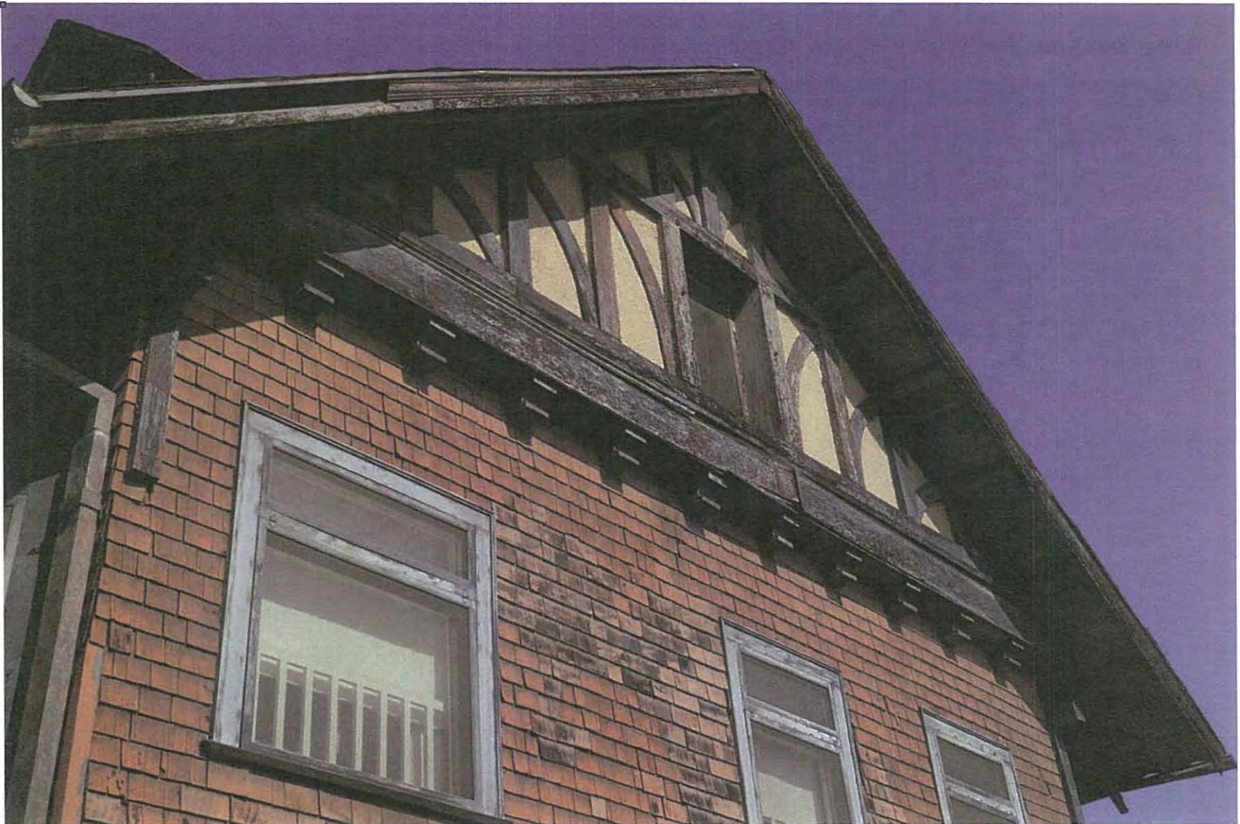
Figure 30 South elevation, detail, second and third stories. Southwest perspective.
