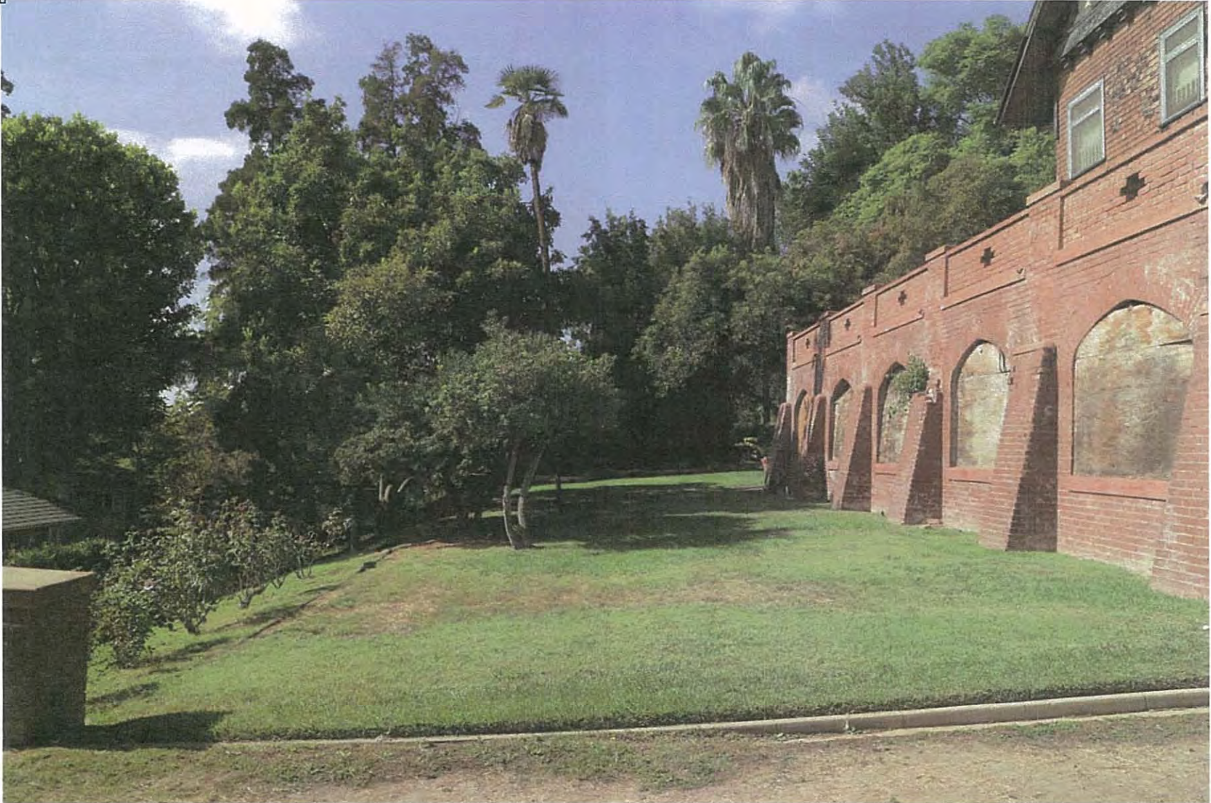
Figure 22 South elevation, exterior walls and buttresses of pool house, and sloping site. Southeast perspective.
