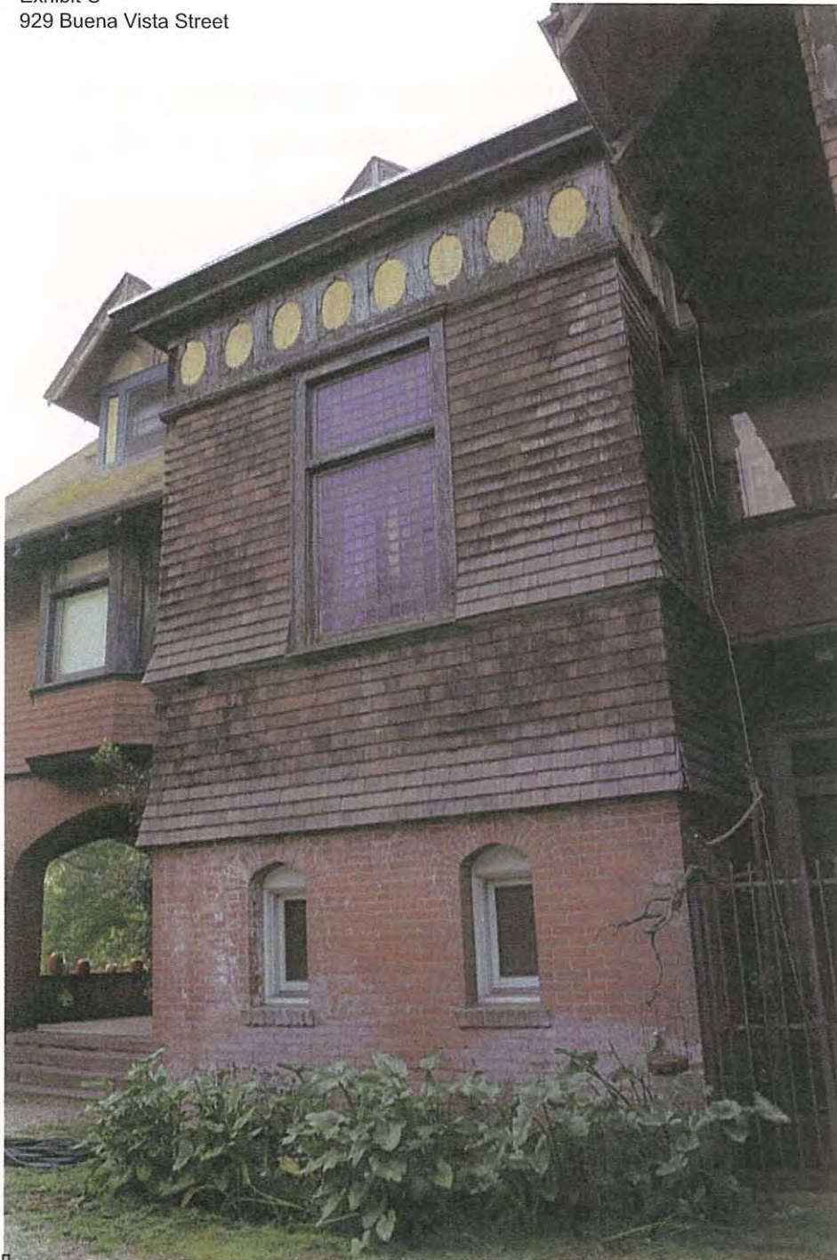
Figure 6 Torrance-Childs Residence, primary elevation, organ tower/confessional detail. Northwest perspective.
