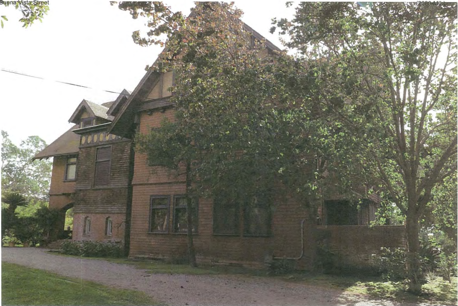
Figure 3 Torrance-Childs Residence, primary elevation. Northwest perspective.
