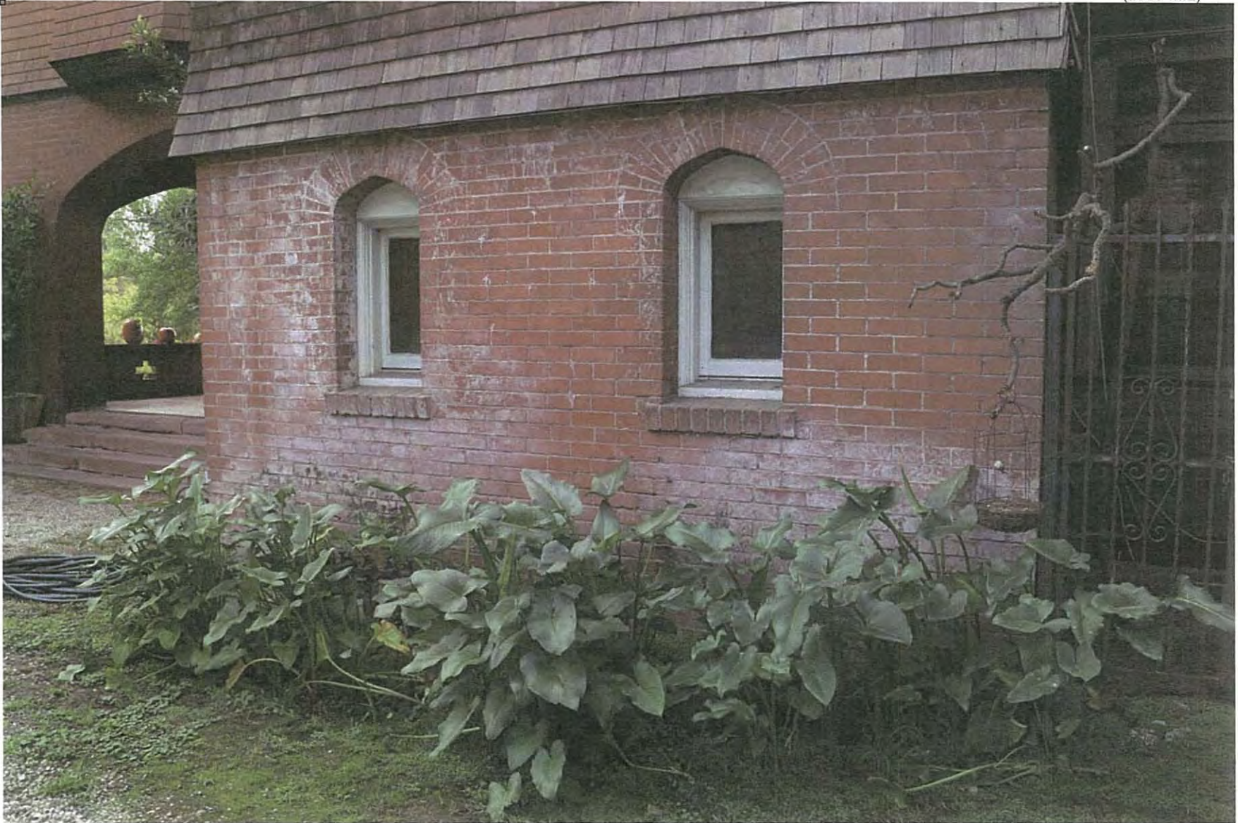
Figure 8 Torrance-Childs Residence, primary elevation. Efflorescence on brick shows areas with water penetration/site drainage issues. Northwest perspective.
