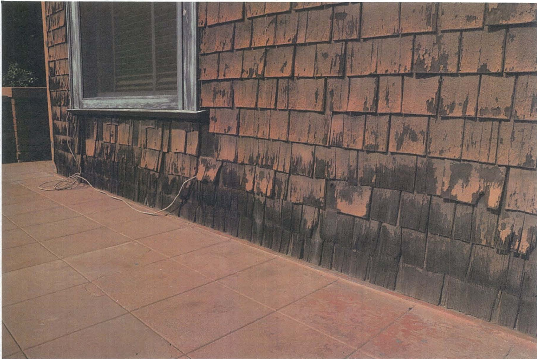
Figure 29 South elevation of residence, from south patio. Example of shingle deterioration. Southeast perspective.
