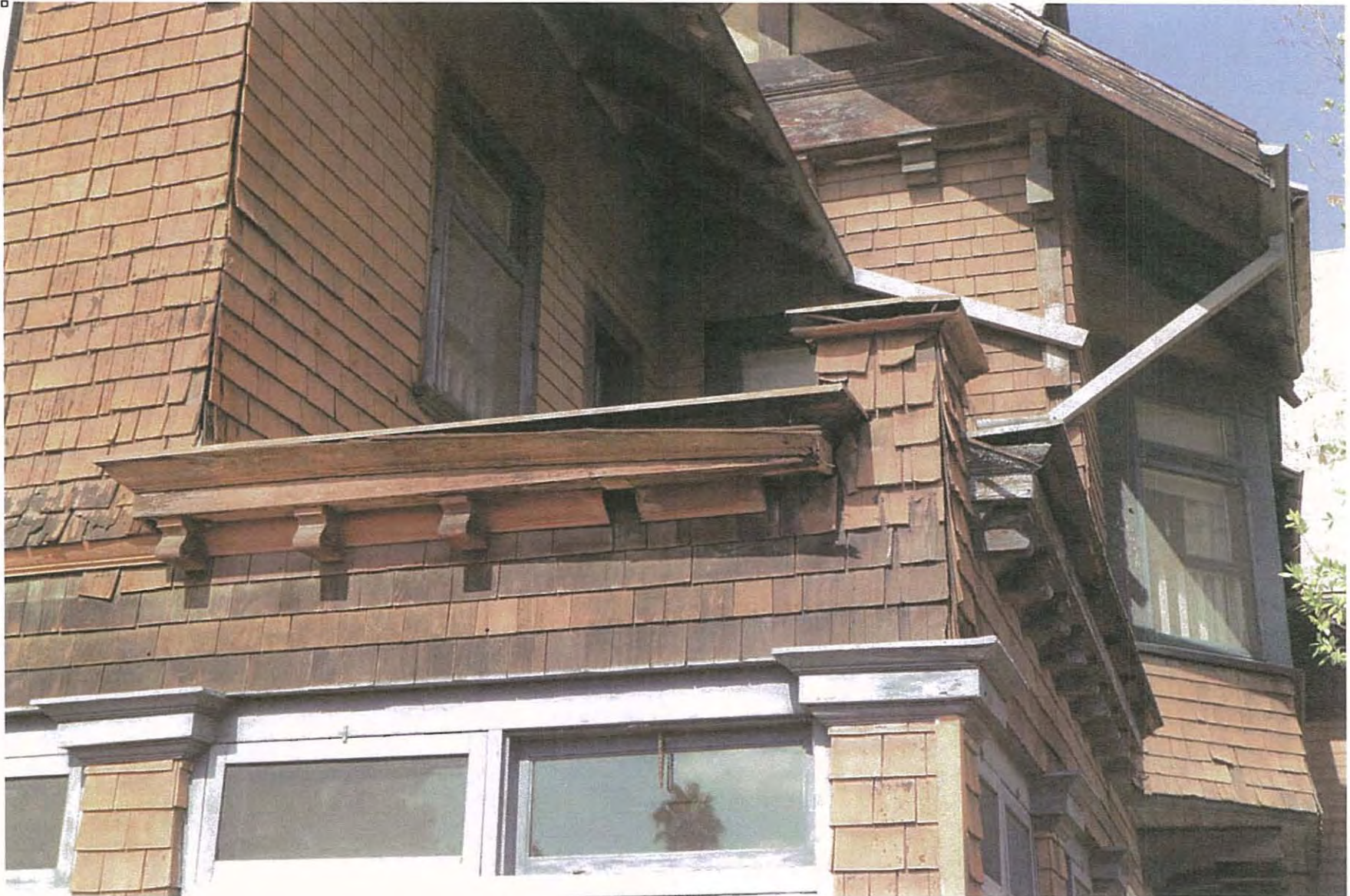
Figure 26 South elevation. Example of carpentry repairs needed. South perspective.
