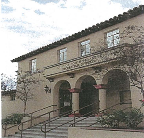
Orange Grove Recreational Building
