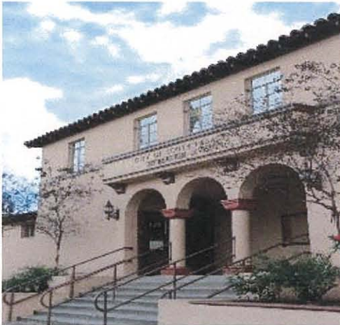
Orange Grove Recreational Building Improvements
