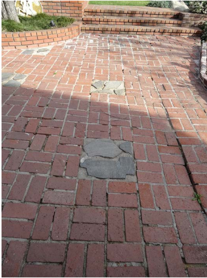
Backyard paving to be restored
