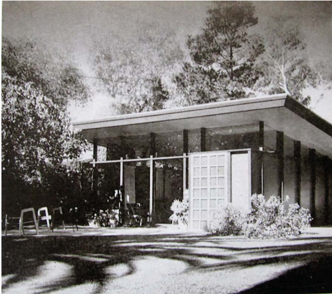
Figure 12 The Smith Residence in 1949, before the façade and living room were extended in 1962. In August 1949, Arts and Architecture published Smith's home, praising it as a "Living Room for a Garden." A month later, the New York Times featured the residence as the illustration for an article entitled "Designs for Better Living, the Home Today and Tomorrow." Source: Arts and Architecture , August 1949.
