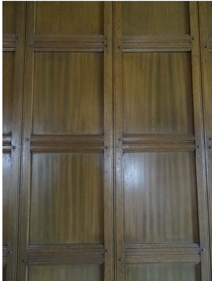
Wood paneling to be restored and waxed
