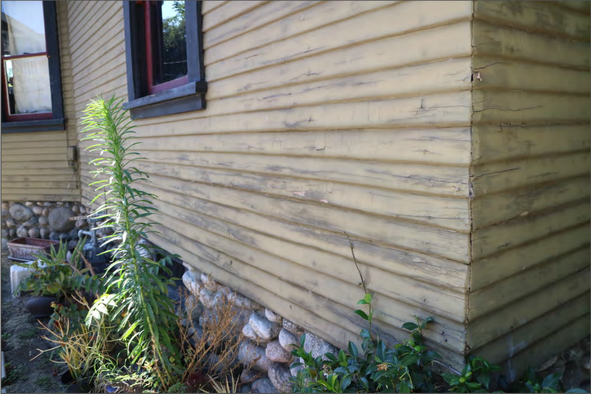
Figure 4. Detail, original horizontal wood-siding, areas in need of repair and repainting
