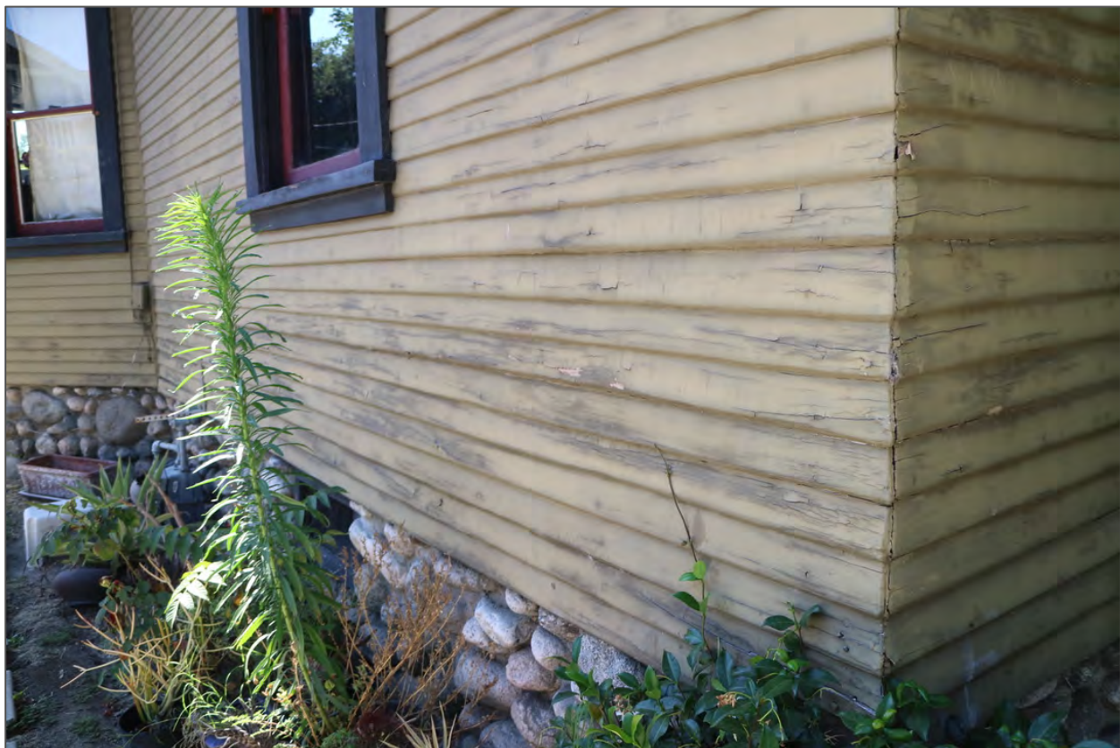
Original horizontal wood-siding, southeast corner of house
