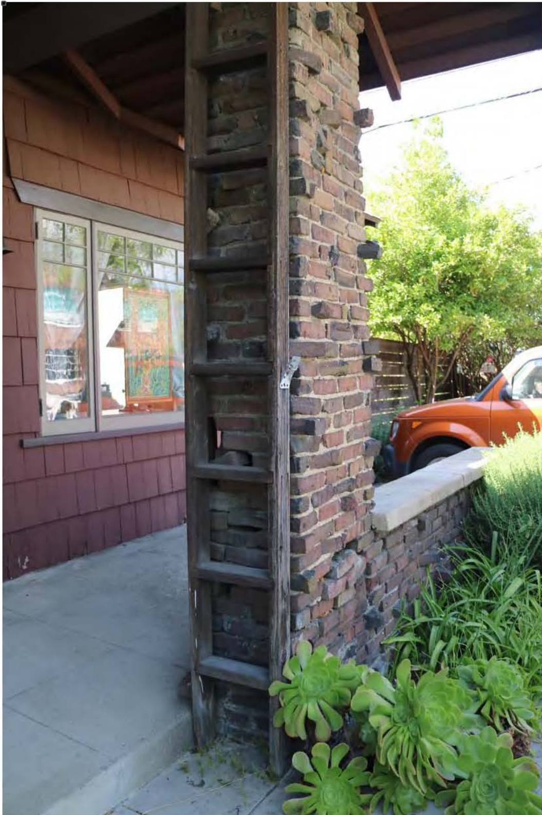
Figure 6. Detail, clinker brick post and temporary wood supports
