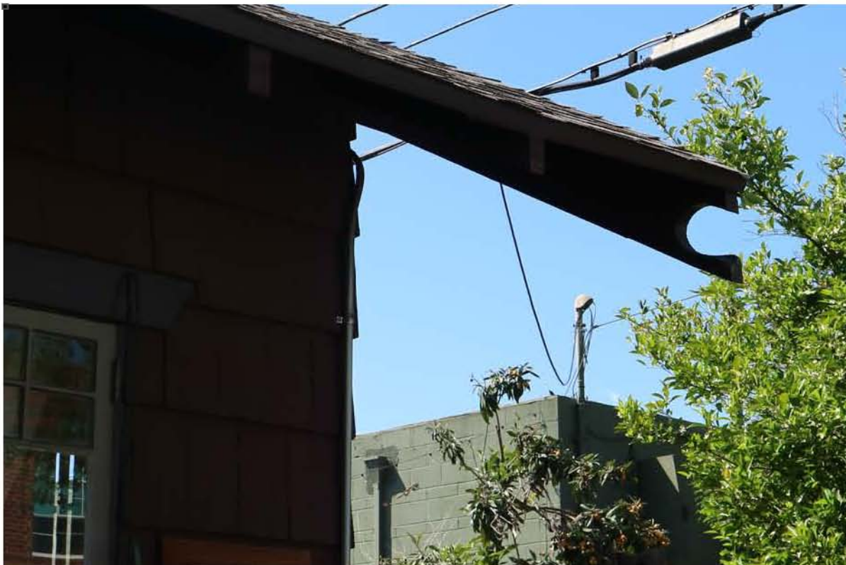
Figure 11. Roof bargeboard and decorative rafter tail to be re-created and repaired
