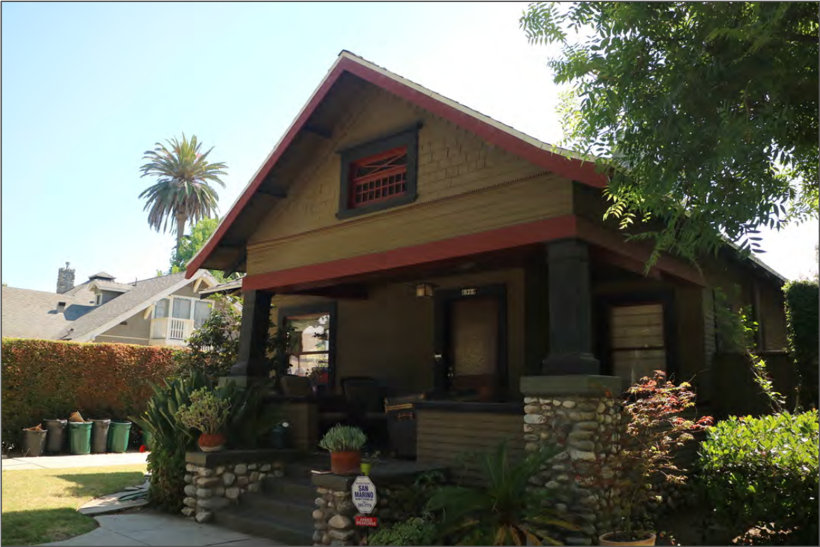
Figure 1. Primary elevation, 925 Palm Avenue (northeast perspective)
