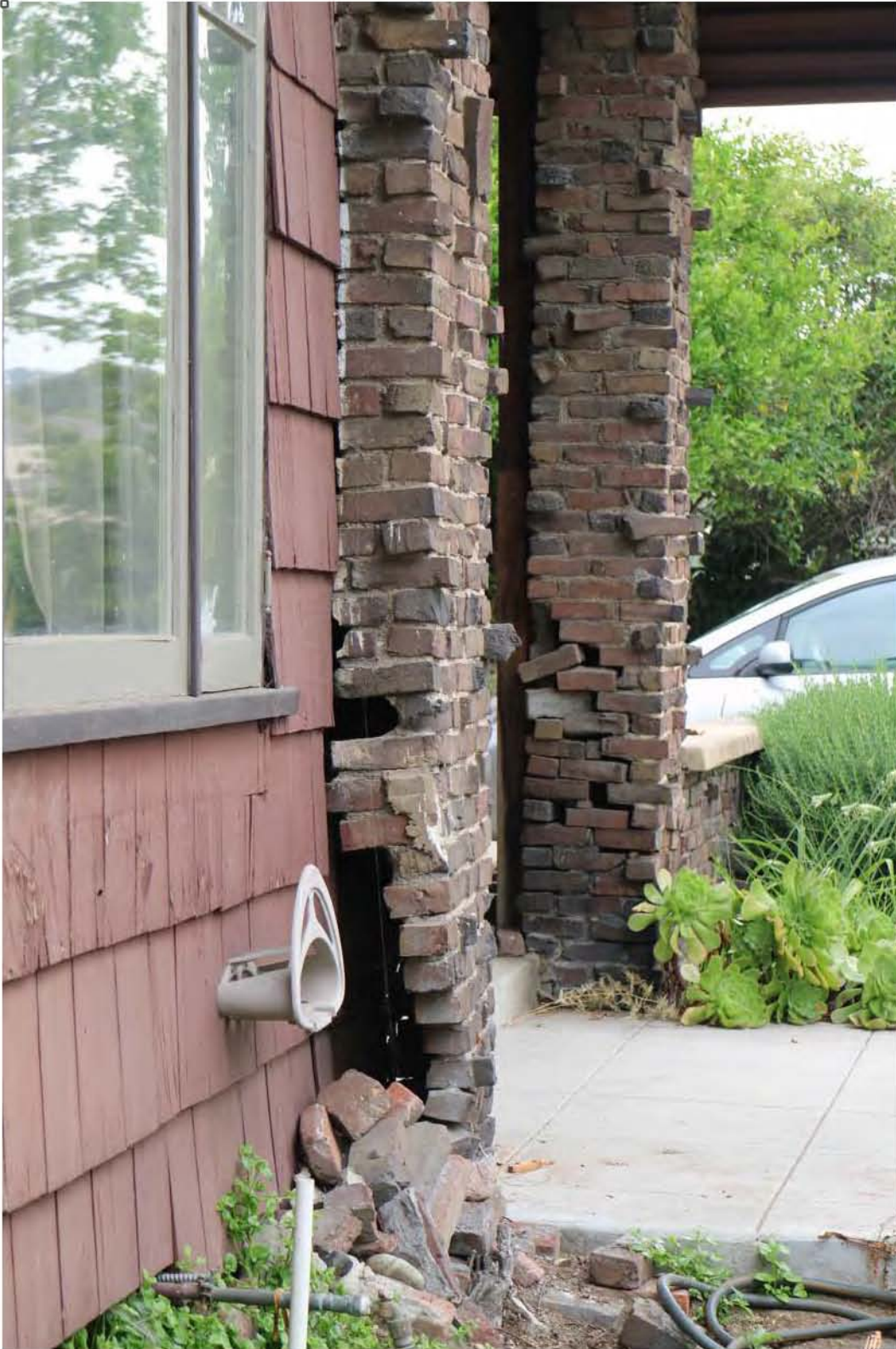
Figure 7. Detail, clinker brick post and temporary wood supports
