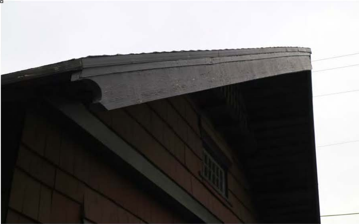
Figure 12. Roof bargeboard and decorative rafter tail to be re-created and repaired
