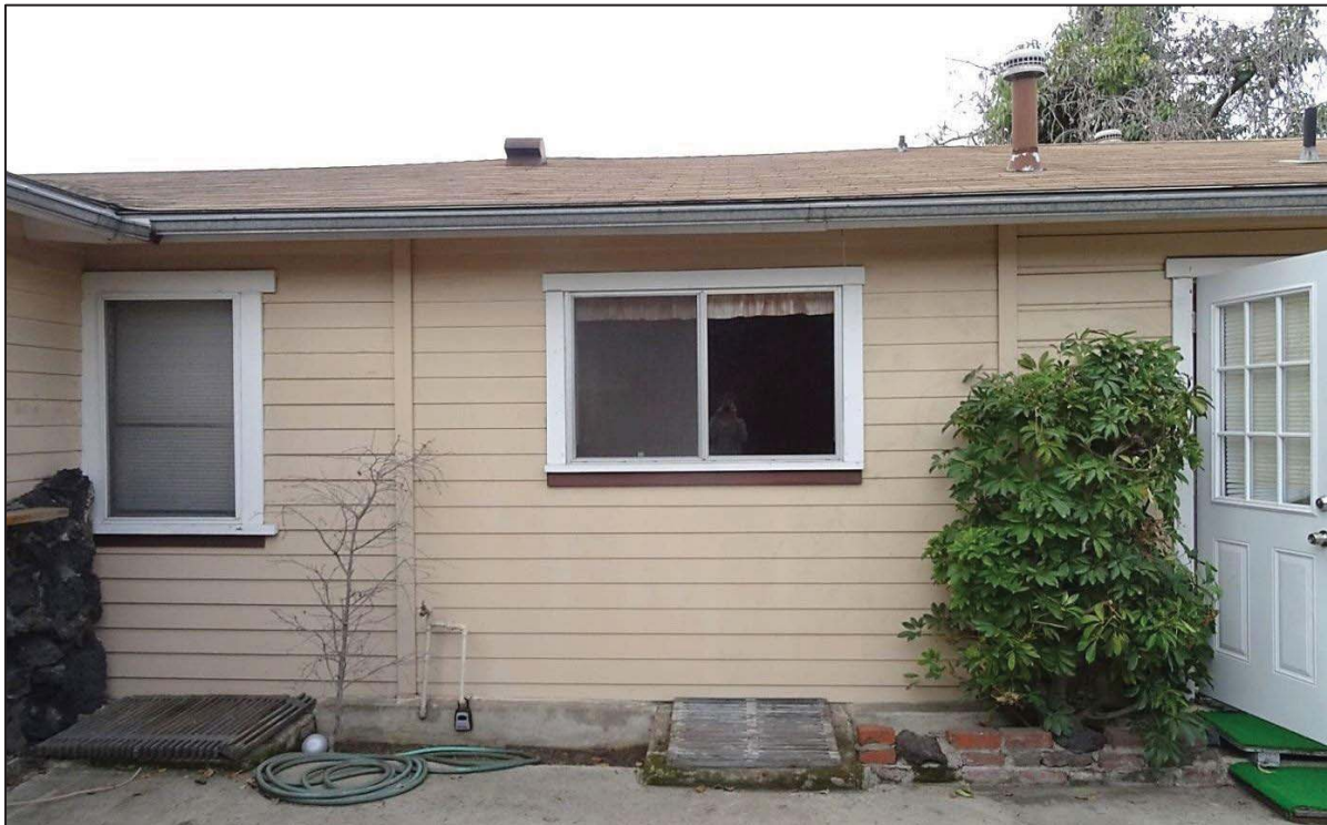
Figure 3 Overview of side (east) elevation, southern portion (top) and northern portion (bottom)
