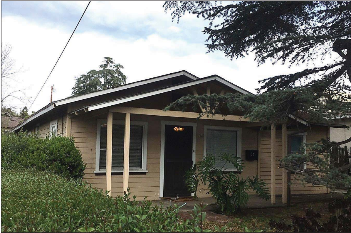
Figure 2 South (façade) elevation, from the southwest (top) and southeast (bottom) perspective, showing addition to property
