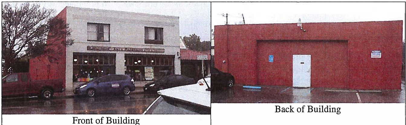
Figure 3: Existing Historic Building
