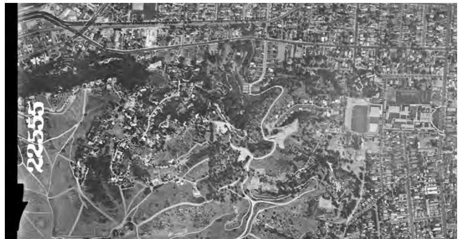
Aerial with Sowards House site work, 1958, UCSB Library Collection
