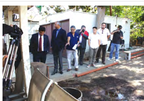
Broken pipes create backyard "Jacuzzi"- Assemblyman Jimmy Gomez [left] and State Senator Roger Hernandez [second from left] inspect the backyard of a home owned by Caltrans where a broken pipe has created what area neighbors refer to as the "Jacuzzi." Randy Economy Photo.
