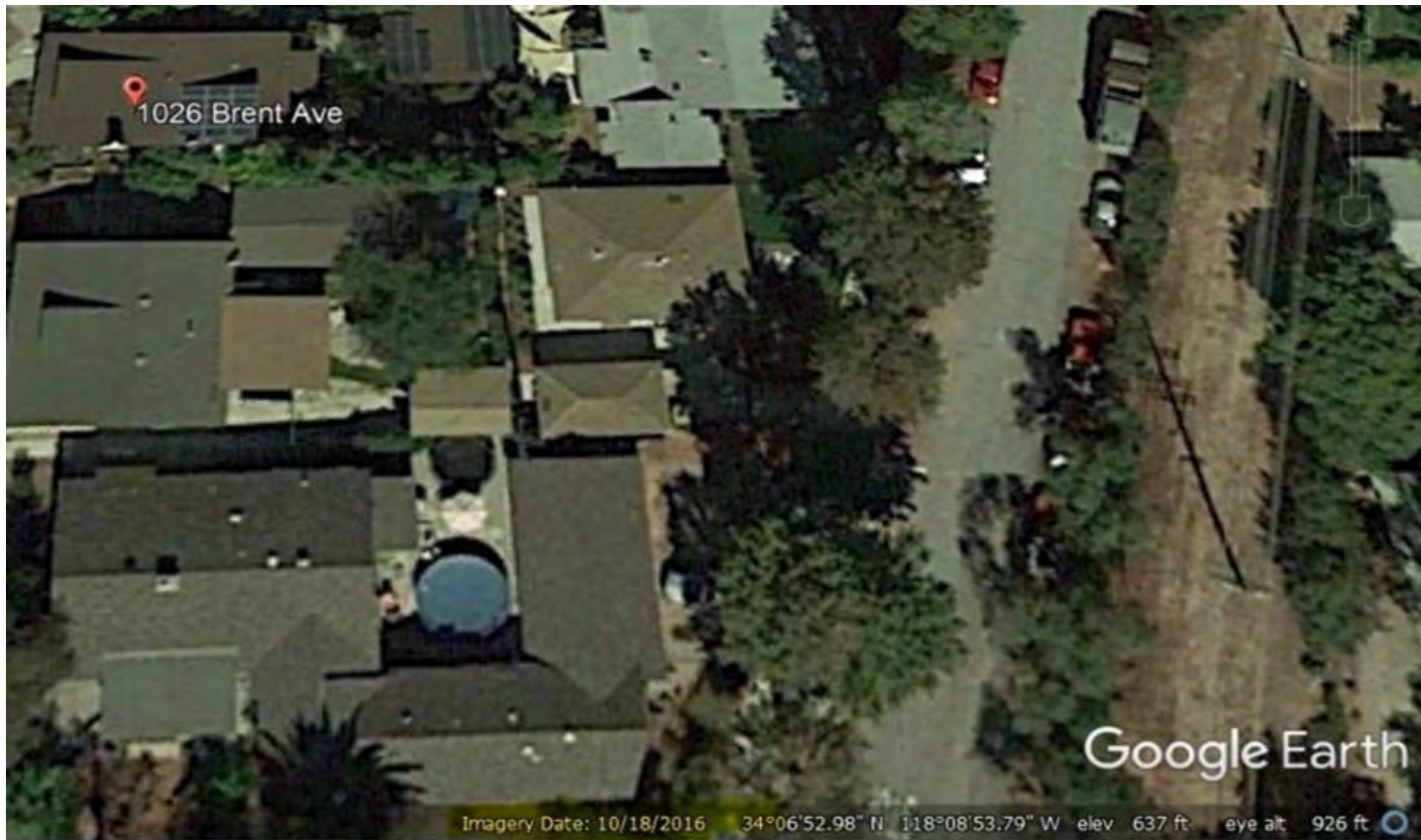
October 2016- flat roof is on and no concrete. 15 months of construction.
