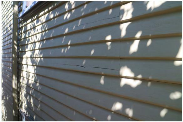
Figure 16. Original horizontal wood-siding on each elevation is in need of repair, gentle sanding/prep work, and repainting
