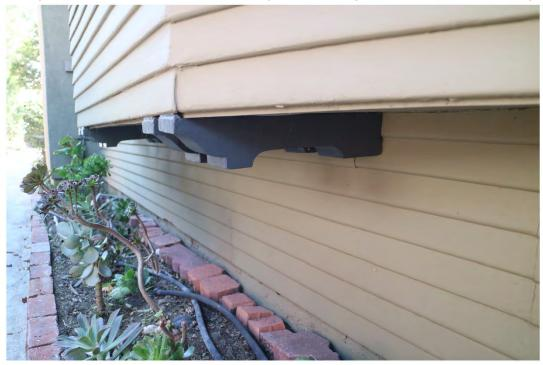
Figure 15. Original horizontal wood-siding on each elevation is in need of repair, gentle sanding/prep work, and repainting
