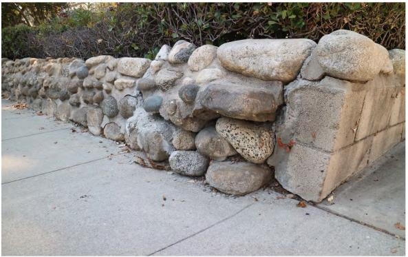
Figure 7. Character-defining hardscaping and stream-rock wall, shows signs of deteriorated mortar and structural failure; in need of repairs, stabilization, and limited in-kind replacement
