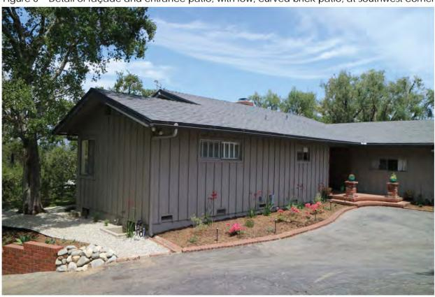
Figure 7 Detail of façade's south-facing wing, with board-and-batten sheathing, minimal fenestration, and brick detailing at entrance
