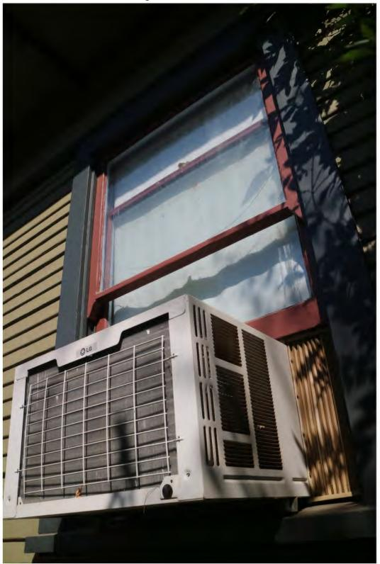
Figure 10. Original wood-frame window, front elevation; some are inoperable, all need repainting of frames and trim and re-weather sealing
