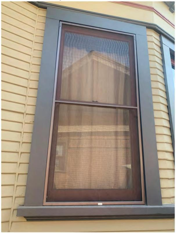
Figure 13. Original wood-frame windows; some are inoperable, all need repainting of frames and trim and re-weather sealing
