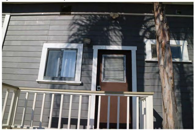
Figure 20 Detail of attenuated, wood-framed two-over-two windows, east elevation
