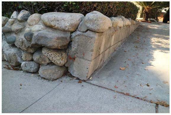
Figure 8. Character-defining hardscaping and stream-rock wall, shows signs of deteriorated mortar and structural failure; in need of repairs, stabilization, and limited in-kind replacement
