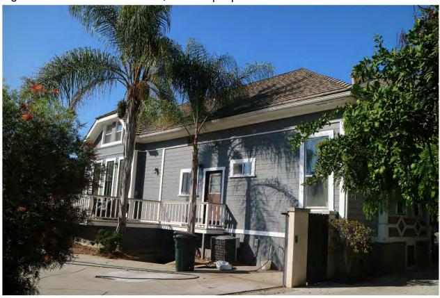
Figure 16 Detail of nonoriginal windows and wall openings, east elevation
