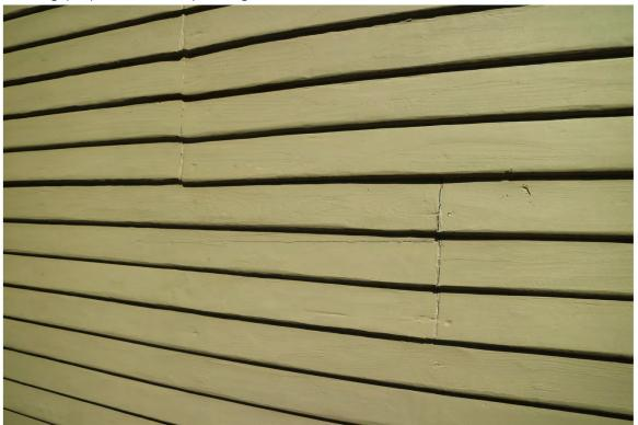
Figure 18. Areas of deteriorated wood siding have been painted over; original horizontal wood-siding on each elevation is in need of repairs/limited in-kind replacement, gentle sanding/prep work, and repainting
