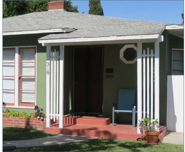
Partial-width projecting porch
