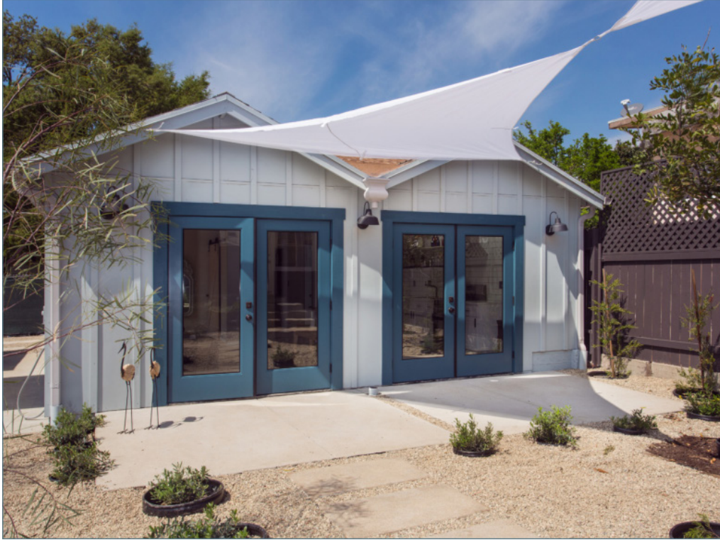
Example of a historic accessory structure conversion (courtesy of Louisa Van Leer Architecture)
