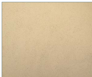
Stucco cladding (sand/float finish)
