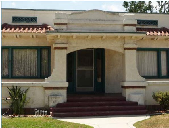
Partial-width projecting porch
