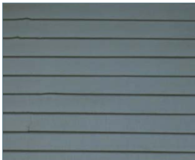
Wood clapboard siding
