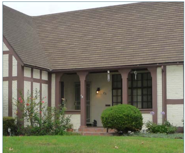
Recessed entrance porch
