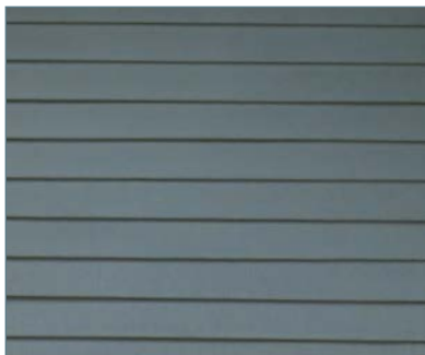
Wood clapboard siding
