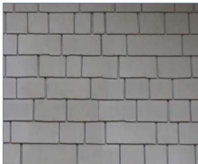
Wood shingle siding (coursed)
