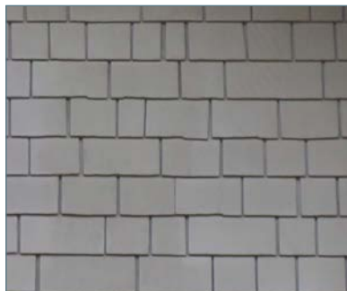
Wood shingle siding (coursed)
