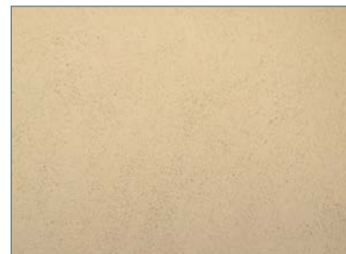
Stucco cladding (sand/float finish)
