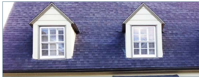
Multiple gable roof dormers
