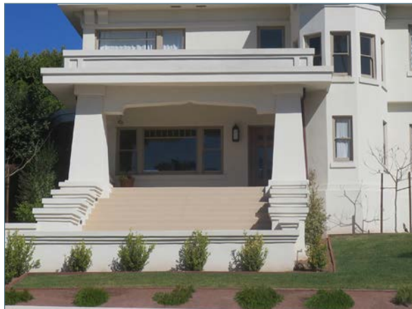
Partial-width projecting porch
