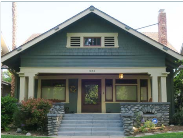
Full-width porch with low stone wall
