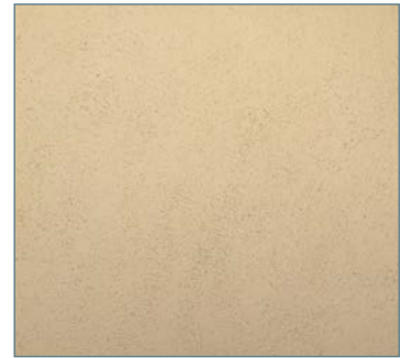
Stucco cladding (sand/float finish)
