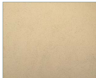
Stucco cladding (sand/float finish)
