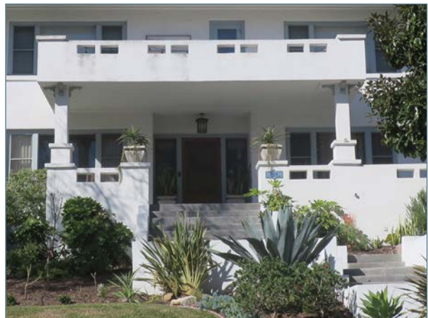
Partial-width projecting porch with low stucco wall
