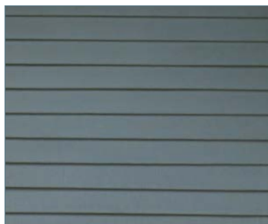
Wood clapboard siding
