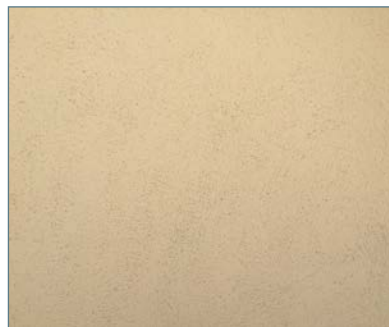
Stucco cladding (sand/float finish)
