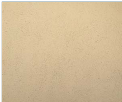
Stucco cladding (sand/float finish)
