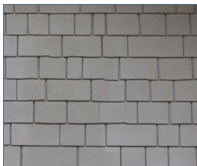
Wood shingle siding (coursed)
