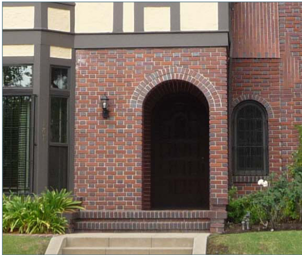
Recessed entrance stoop
