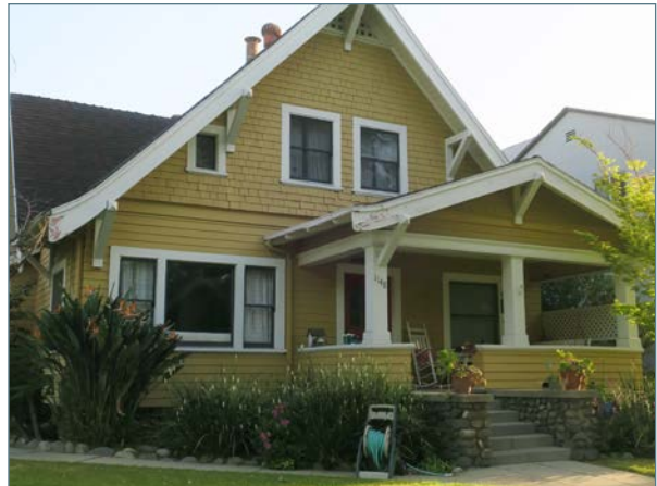
Partial-width projecting porch with wood knee wall
