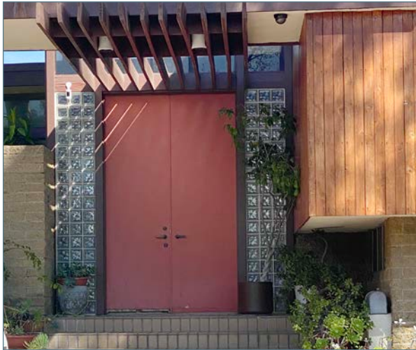
Recessed entrance stoop
