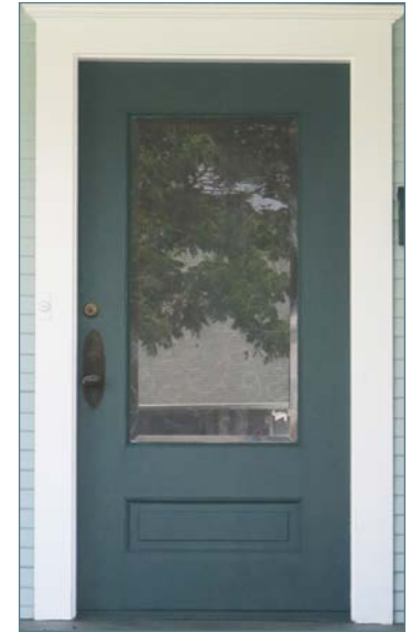
Paneled wood door with glazing
