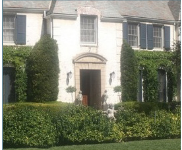
Recessed entrance stoop
