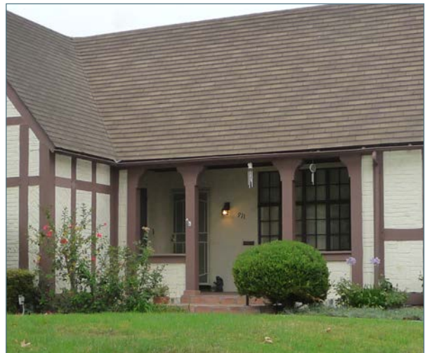
Recessed entrance porch
