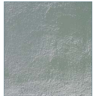
Stucco, sand/float finish
