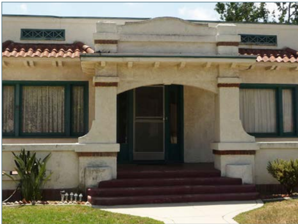
Partial-width projecting porch
