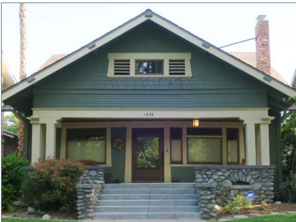
Full-width porch with low stone wall
