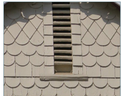
Wood shingle siding (variegated)
