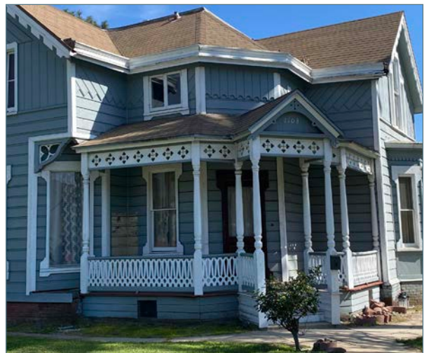
Wraparound porch with wood railing
