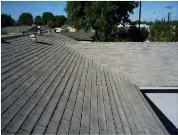
Roofing Shingle in fair condition
