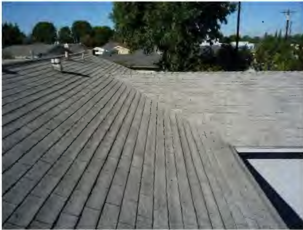
Roofing Shingle in fair condition
