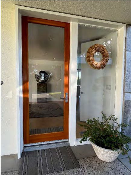
Front door to foyer (P14)
