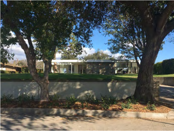
Street view, elevated behind retaining wall (P1) 2
