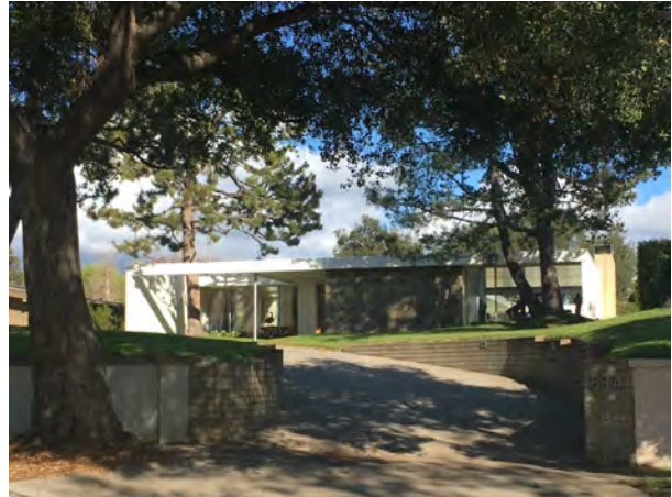
Driveway to front façade (P2)
