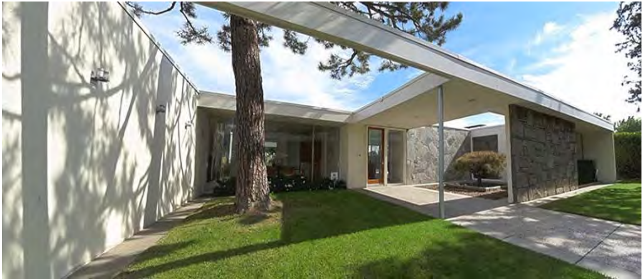
Cox Residence. Photograph credit: georgearchitecture.com
