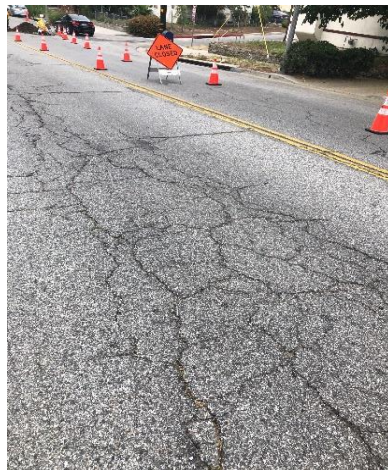
Description: Block Cracking at Monterey Road
