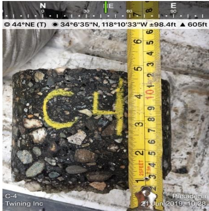
Description: C4 – EB Monterey Rd - 117ft E/O Brunswick Ave
