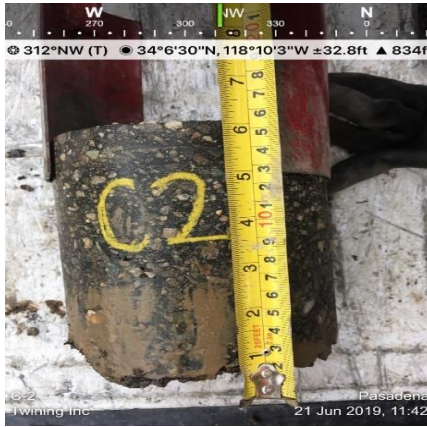
Description: C2 – SB Alta Vista Ave - 140ft W/O Mountain View Ave
