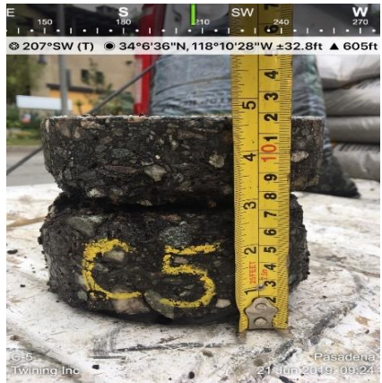
Description: C5 – WB Monterey Rd - 194ft E/O Kolle Ave
