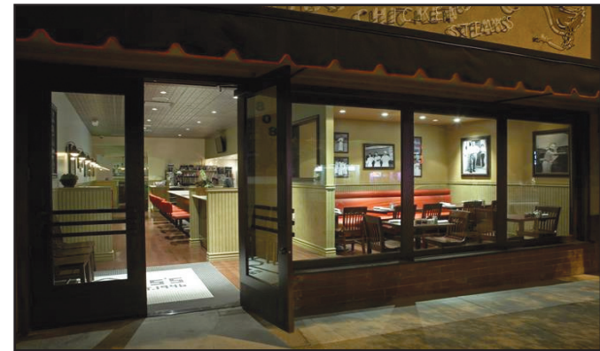
Brick, tile and stucco are traditional storefront materials
