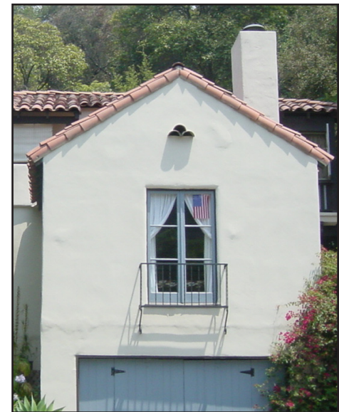
Stylized attic vent and metal railing
