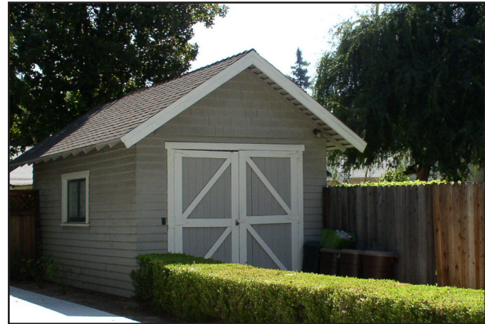
Secondary structure with siding, roofing detailing consistent with the primary residence.
