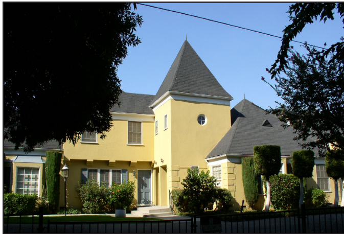
This house has asymmetrical massing often found in this style.
