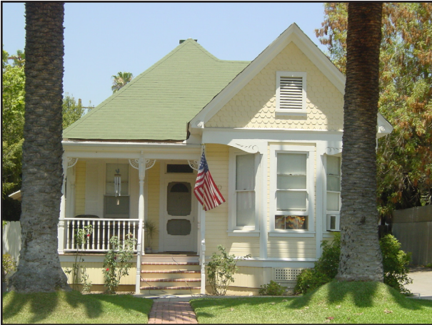
This small cottage has Queen Anne detailing including shingled gable face, bay window and turned porch railings.
