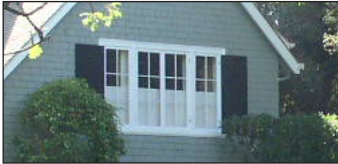
True divided light wood windows, often grouped in pairs or bays are typical; shutters are common on some styles.
