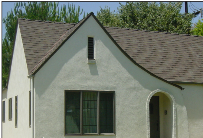
Stucco with a smooth finish was used historically.
