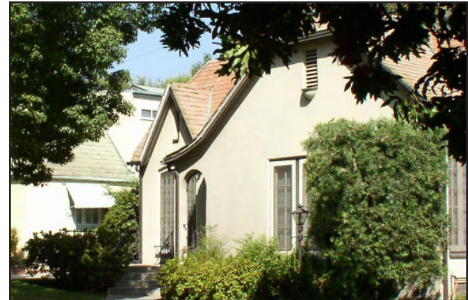
Curved rooflines at the entry is a common feature.
