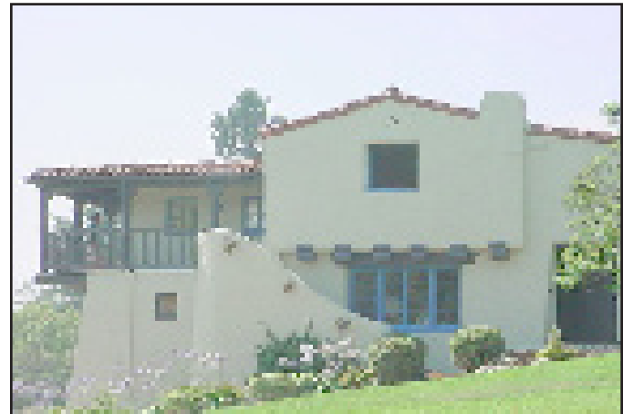
Spanish Colonial Revival houses with red tile roof, exterior stairway, overhanging porch and smooth-troweled stucco finish.
