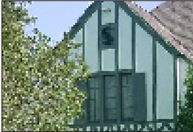
Stucco with half-timbering on a Tudor style house.
