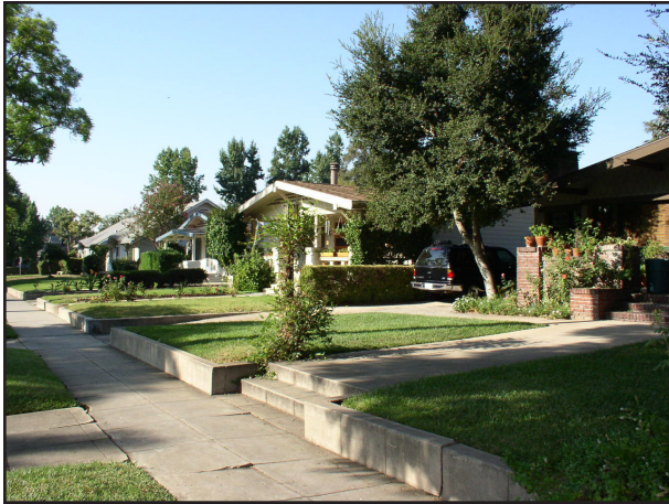
Historic concrete retaining walls, stairs, sidewalks, and walkways.
