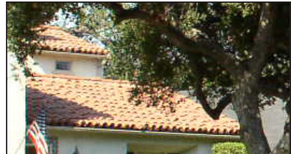
Clay tile roof.
