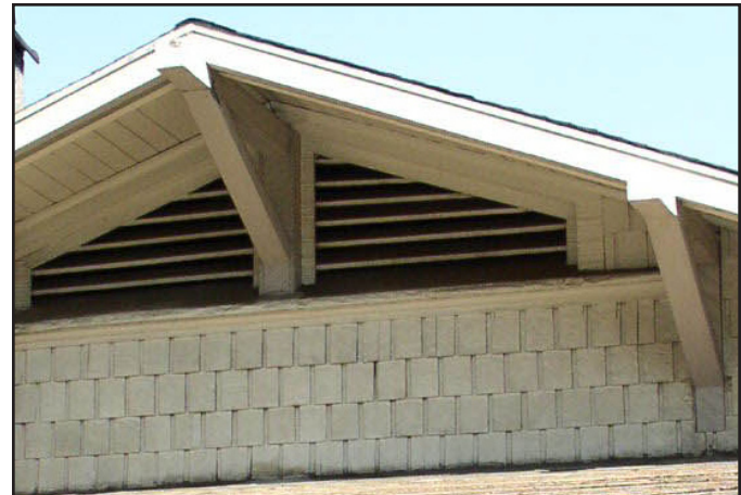
Wood shingles at gable eaves.
