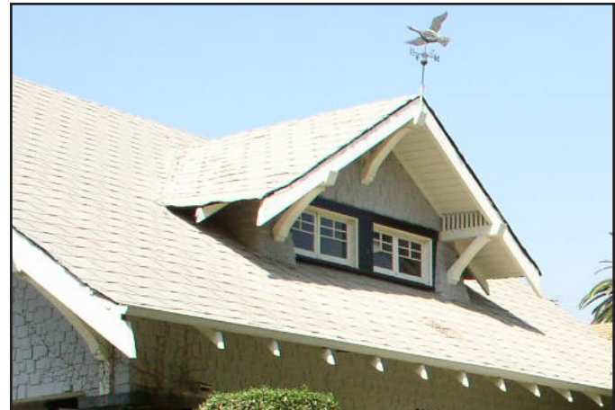
Composition shingles on a Craftsman style roof and dormer.
