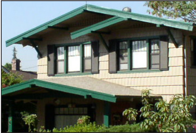
Typical low sloping gable roofs with large overhangs on a Craftsman Style house.
