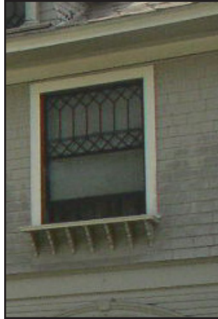
Wood windows with single glazing and true divided lites.
