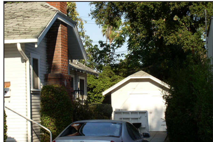
Secondary structure with roof form, materials and detailing that match the house.
