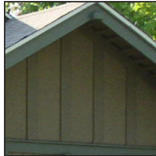
Wood board and batten
