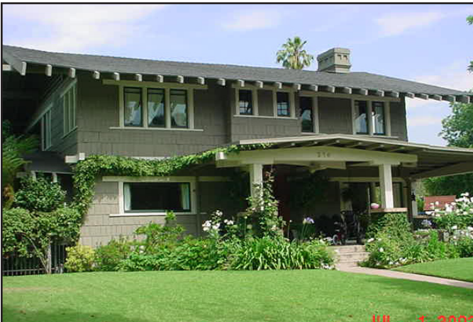
Overhanging eaves with exposed rafter tails are common on Craftsman houses.
