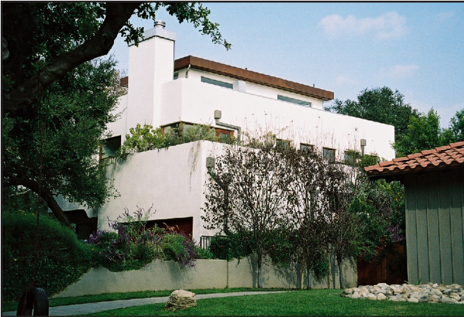
This house has Modern elements including smooth stucco walls and limited decoration.
