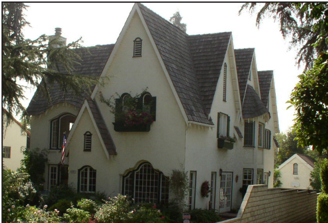
Typical steeply sloped roof forms with wood shakes on a Tudor Revival house.
