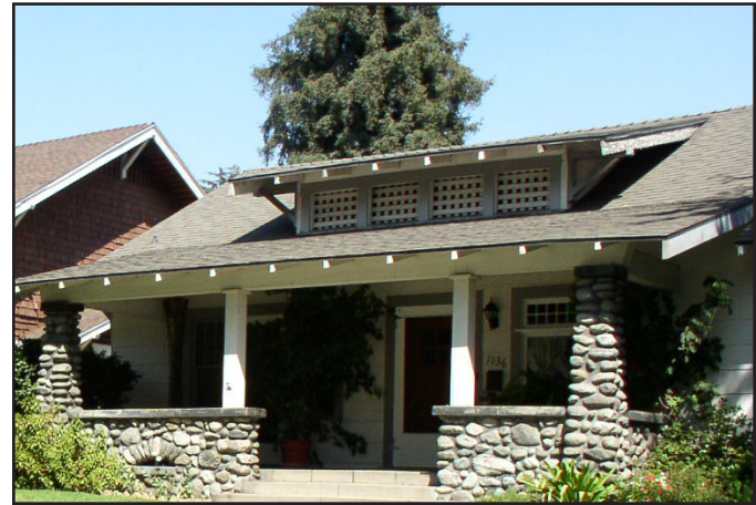
Craftsman Bungalow with battered piers
