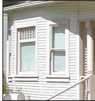
Wood clapboard siding
