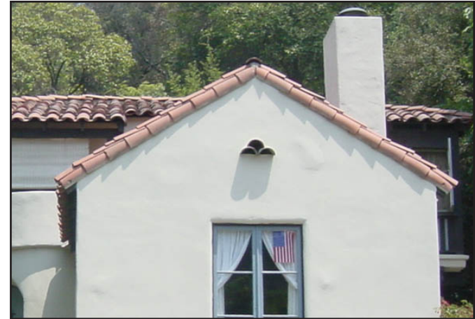
Decorative coping of red tile at the eaves and ceramic vents at the gable are often employed.
