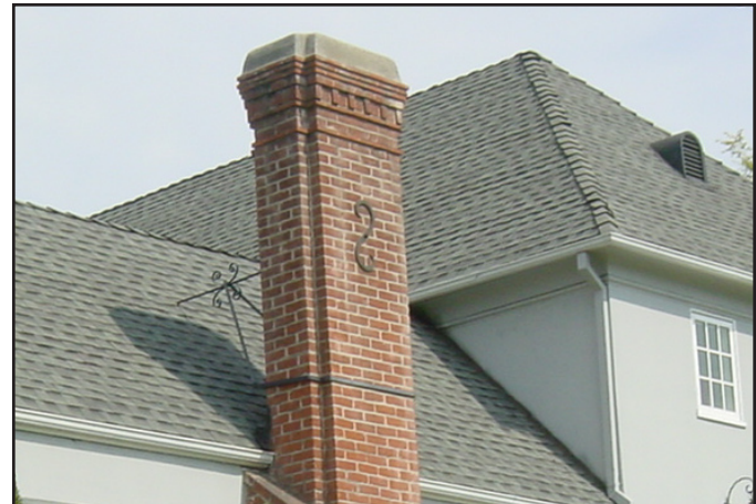
Brick chimney projecting from the roof line of this house.
