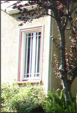
Wood windows with single glazing and true divided lites.
