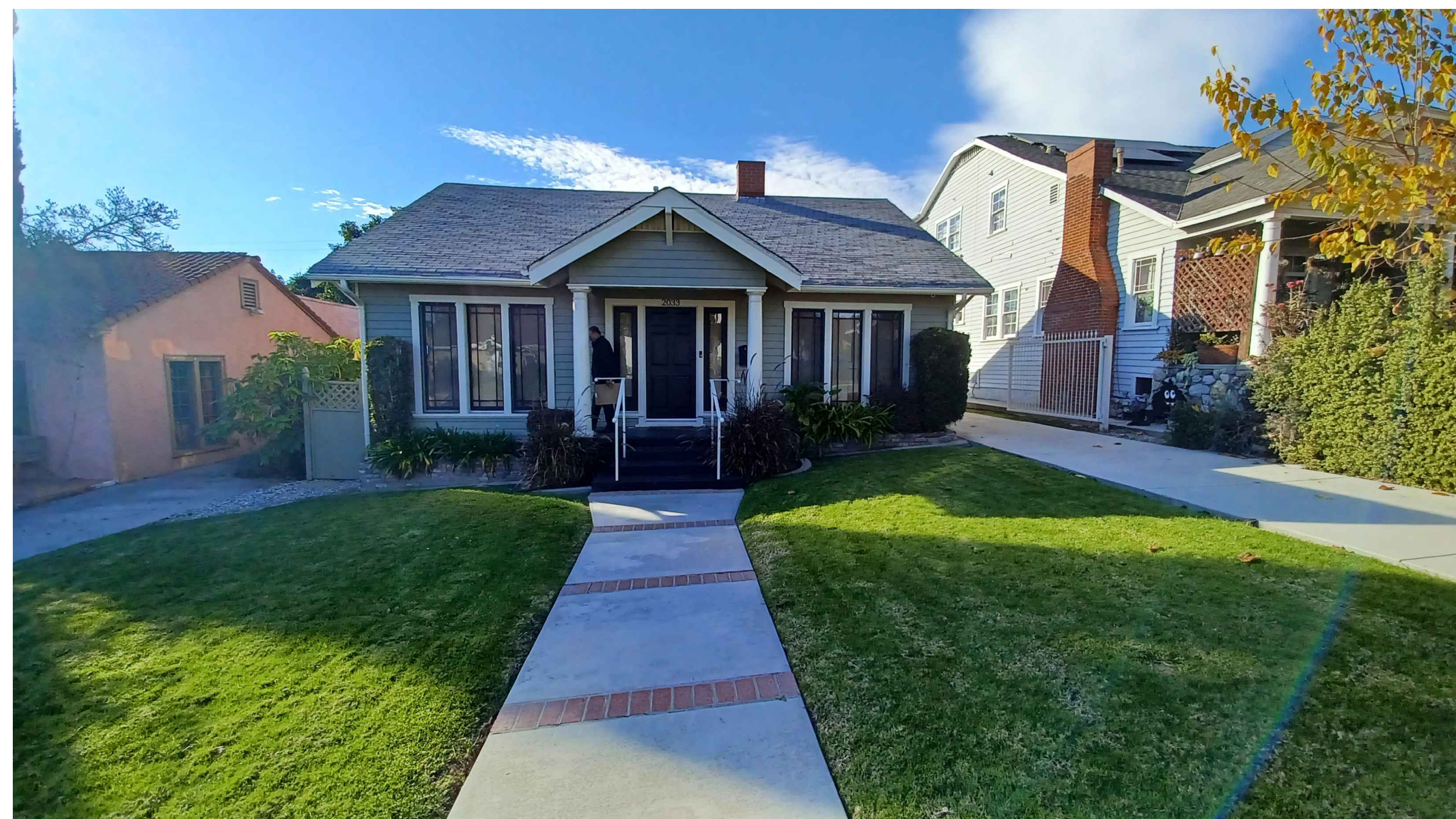
2033 ALPHA AVE. BEFORE CHANG RESIDENCE
