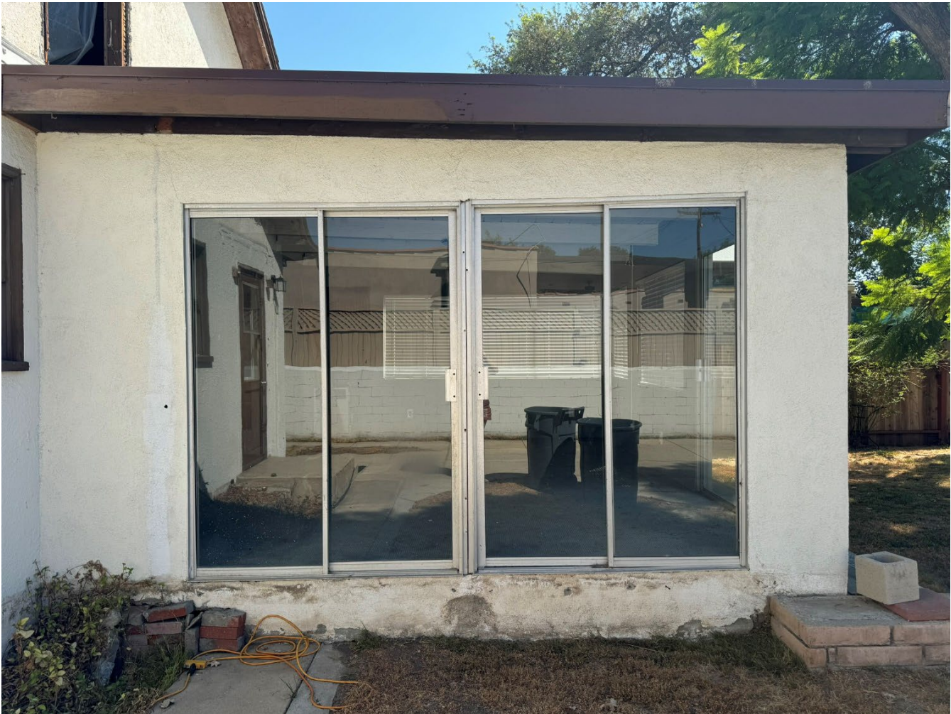
Existing Windows to be Removed/Replaced
