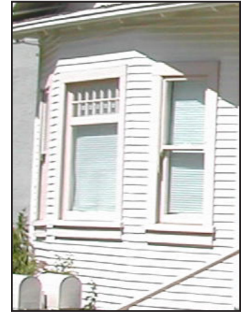
Wood clapboard siding
