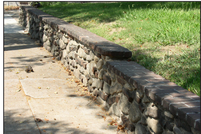
Retaining walls of varying materials are also found in South Pasadena.
