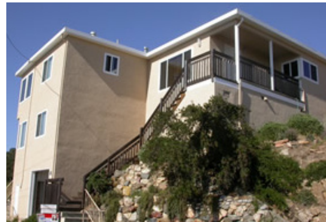
This hillside residence fails to create an engaging facade. The placement of the windows and plain stucco wall does not offer an interesting facade arrangement.
