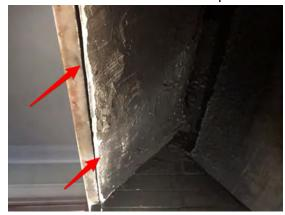
There are combustible materials on the facing which violate the code for the clearance to combustibles. Although this is a code violation there did not appear to be any damage due to this.
