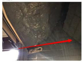
The required lintel is missing. This can allow premature damage to the masonry structure above the opening and the facing. A lintel will need to be installed
