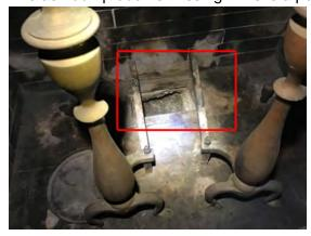
The walls in the firebox sound loose or hollow when knocked upon. This is an indication that the firebox lining is no longer protecting the structural walls of the chimney.
