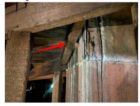
During the attic inspection evidence of water intrusion was noted on the framing members around the chimney stack. Flashing issues found have been noted in this report.
