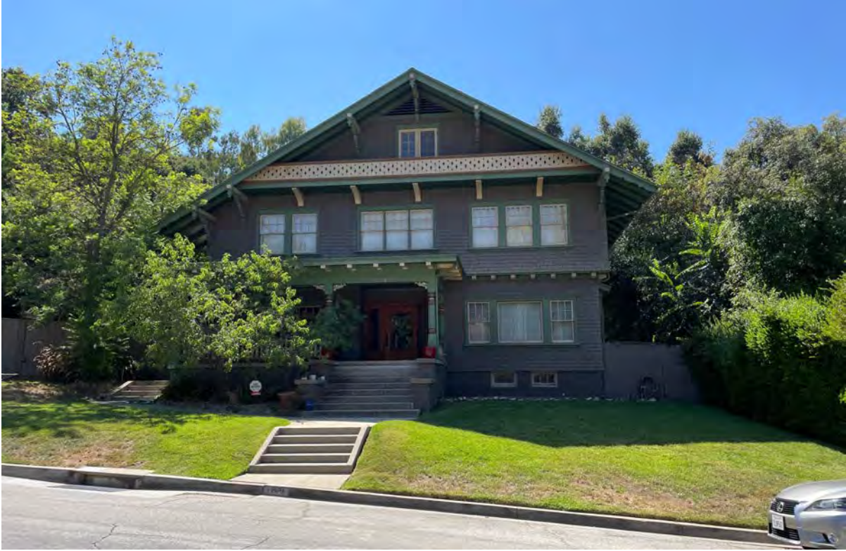
Figure 3 Overview of façade, east perspective
