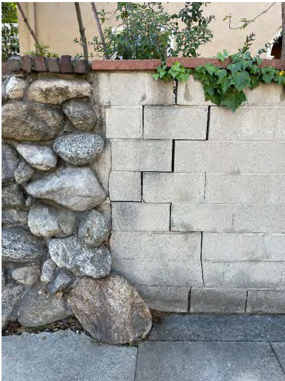
Block walls and Arroyo stone posts to be repaired
