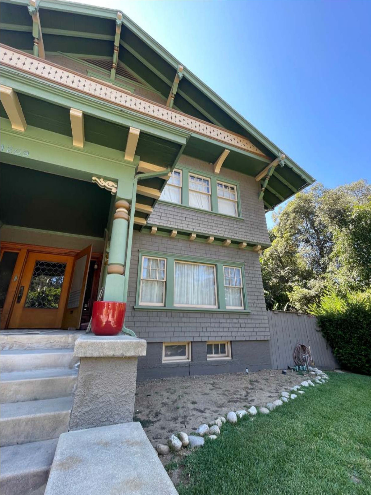
Figure 6 Façade detail, east perspective
