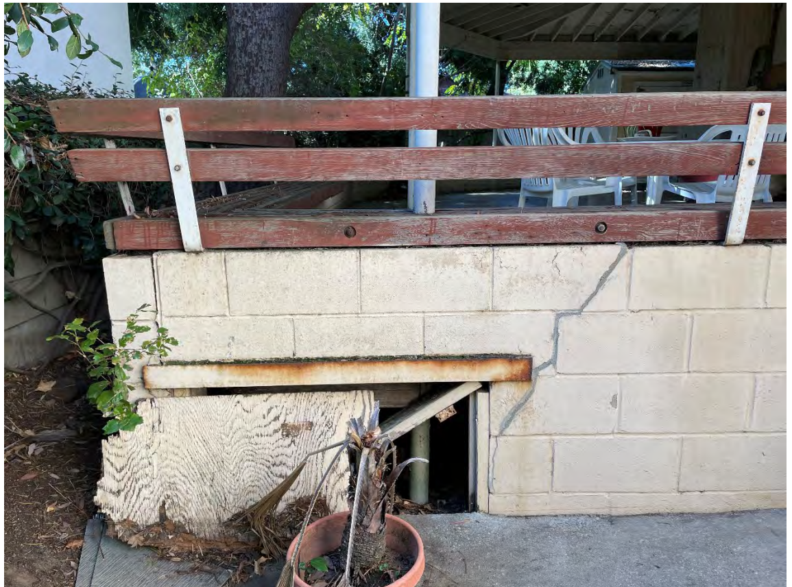
Attached rear porch – roof and foundation damage
