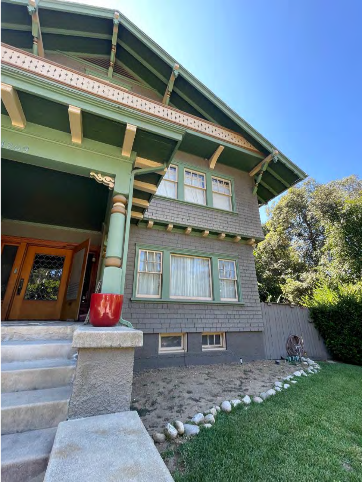
Figure 6 Façade detail, east perspective
