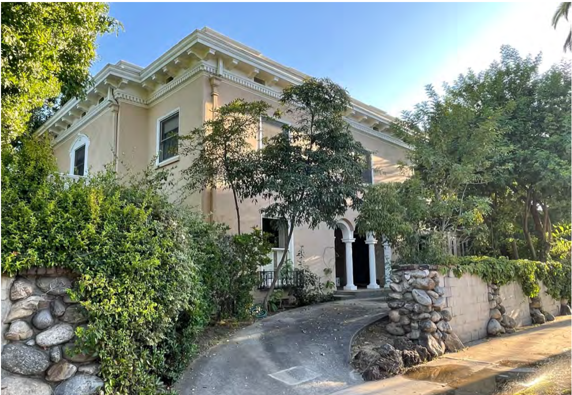
203 Oaklawn Ave, side (north) elevation
