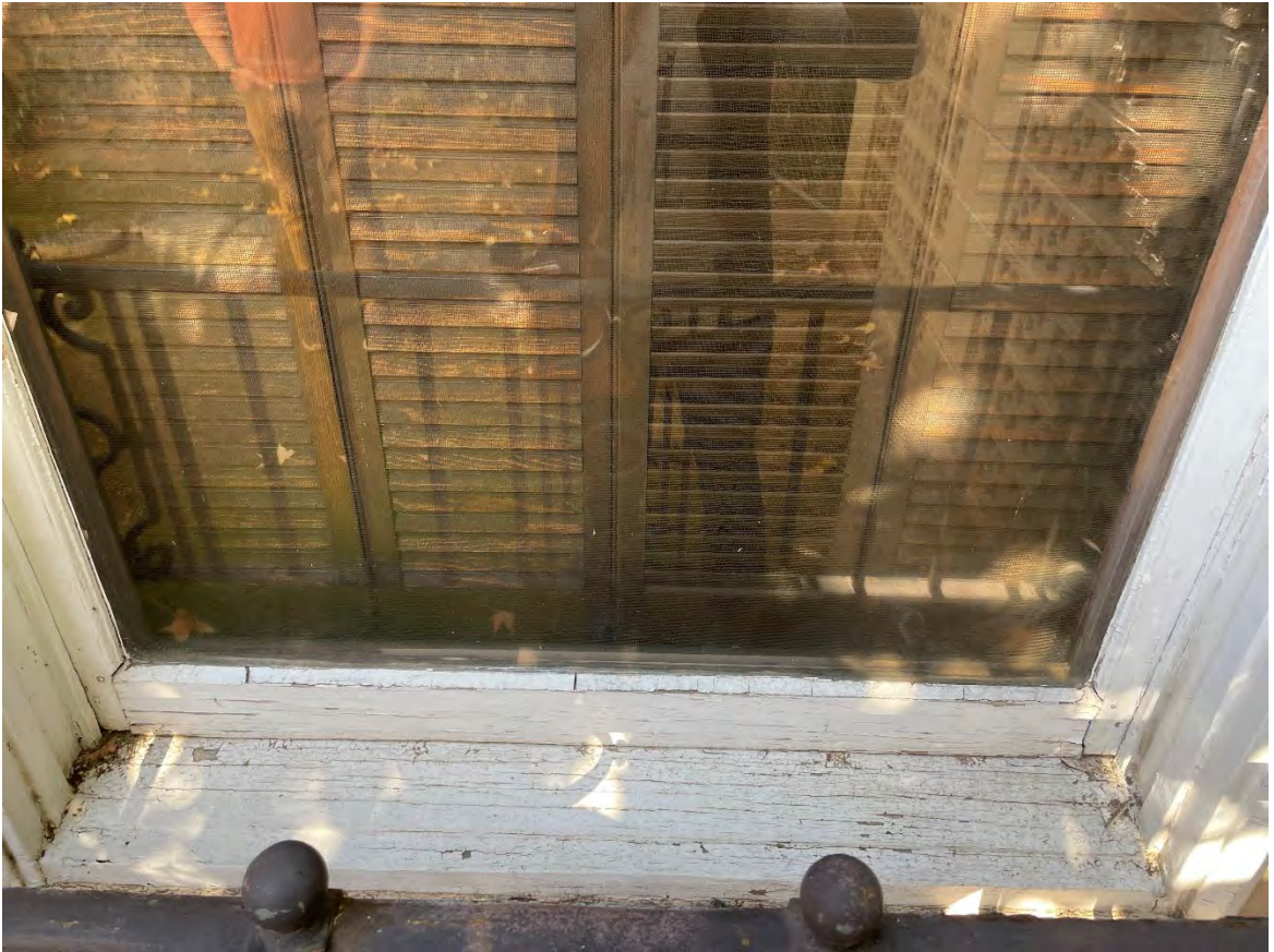
Deteriorated original windows with cracks and peeling paint
