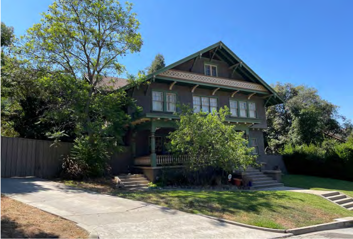
Figure 4 Overview of façade, southeast perspective
