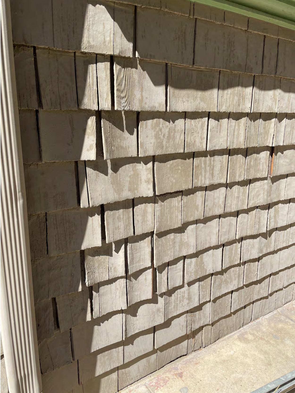
Figure 15 Detail of wood shingles, south elevation, southwest perspective
