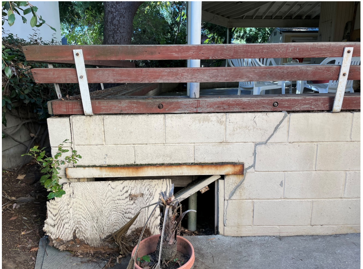
Attached rear porch – roof and foundation damage
