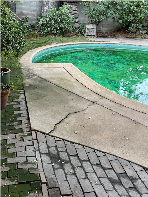
Clinker brick pavement to be repaired
