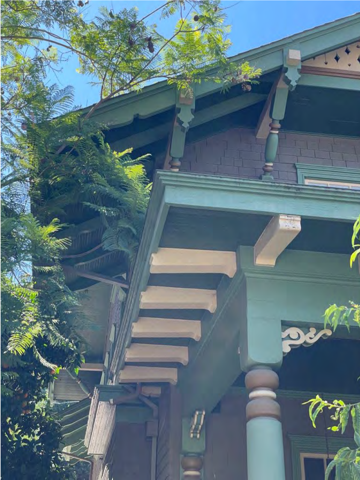
Figure 9 Detail of roof detailing and entrance porch, east perspective
