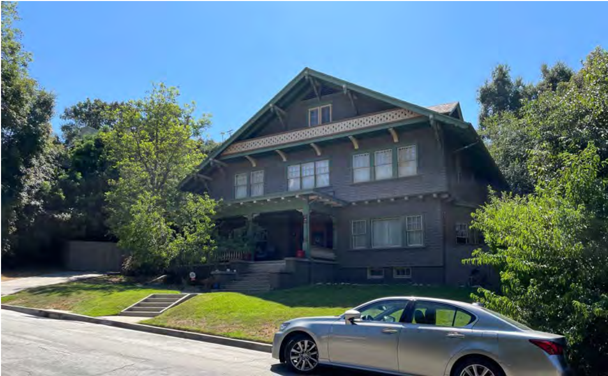
Figure 2 Overview of sloped, hillside parcel, façade, northeast perspective
