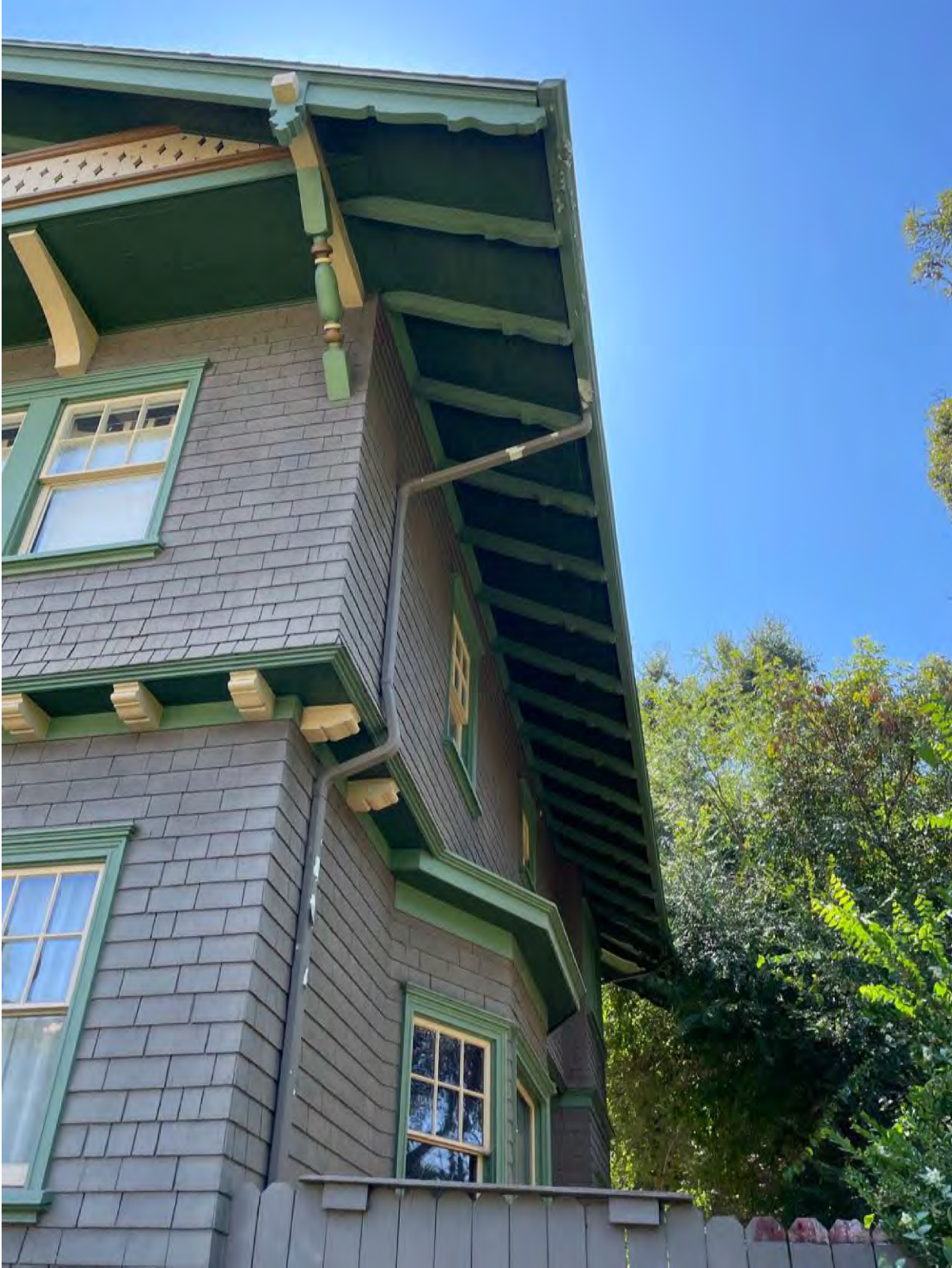
Figure 13 Corner of east and north elevations, northeast perspective
