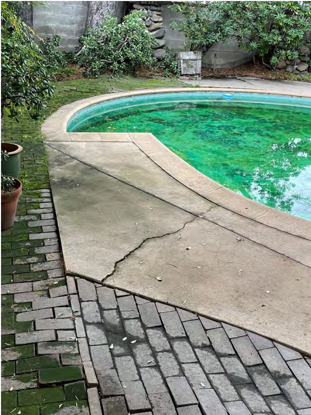
Clinker brick pavement to be repaired
