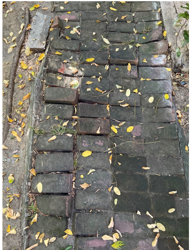
Clinker brick pavement to be repaired
