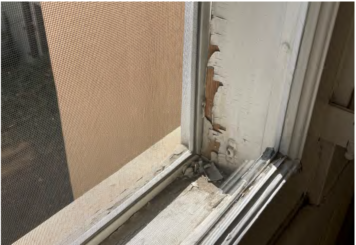
Deteriorated original windows with cracks and peeling paint
