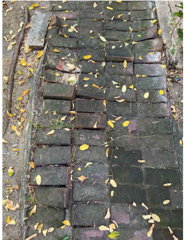
Clinker brick pavement to be repaired
