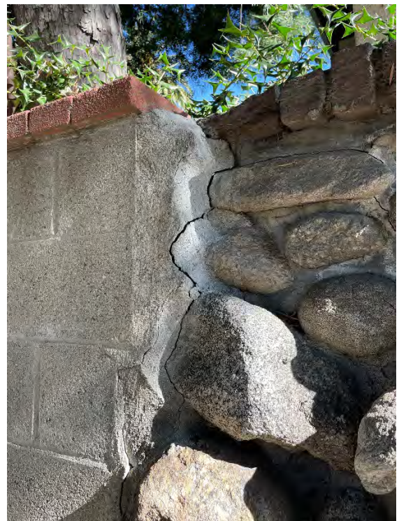
Block walls and Arroyo stone posts to be repaired
