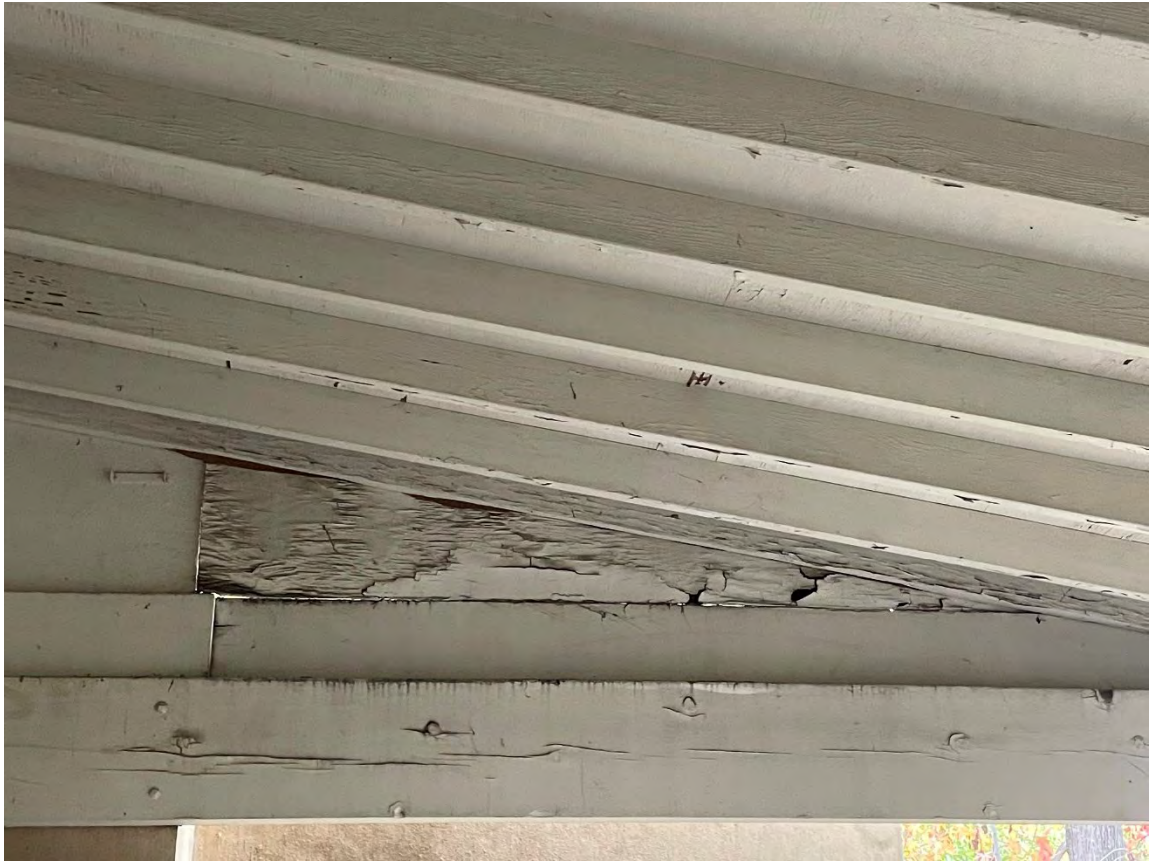
Attached rear porch – roof and foundation damage
