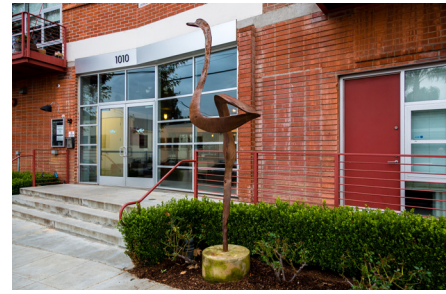
Creative office building (Class B, 102,660 s.f.) in Ostrich Farm area, built in 2006
