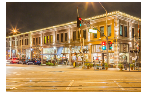
Mixed-use building on Mission Street designed in "commercial vernacular" style with minimal decorative detailing.
