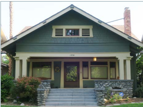
Full-width porch with low stone wall
