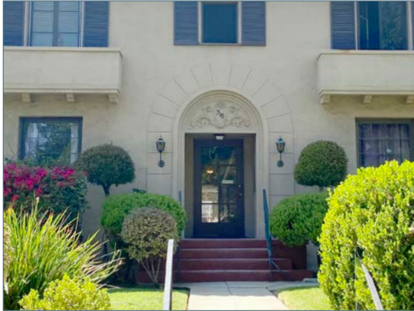
Recessed entrance stoop
