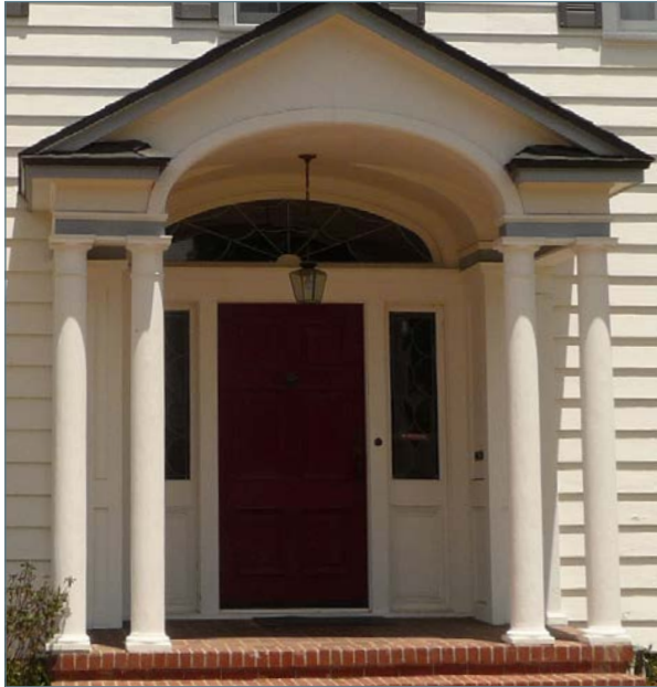
Projecting entrance stoop
