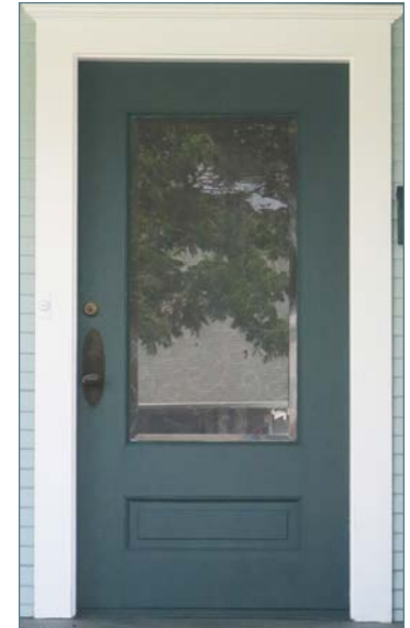
Paneled wood door with glazing
