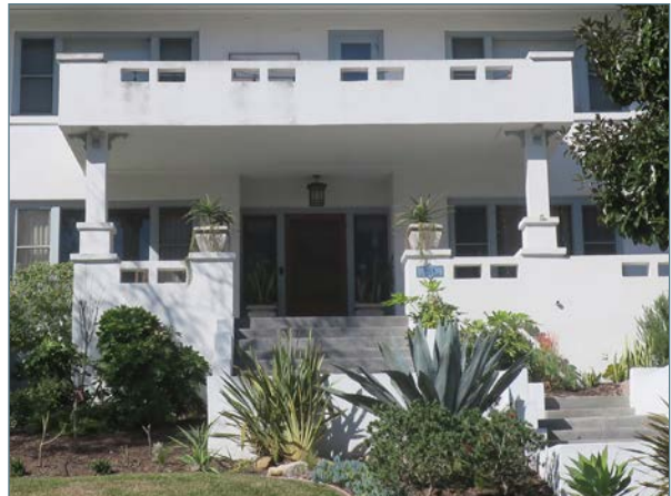
Partial-width projecting porch with low stucco wall
