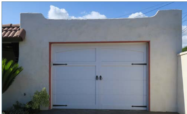
Existing (non-historic) garage doors on accessory structure
