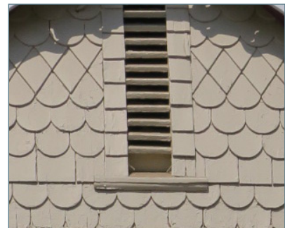
Wood shingle siding (variegated)
