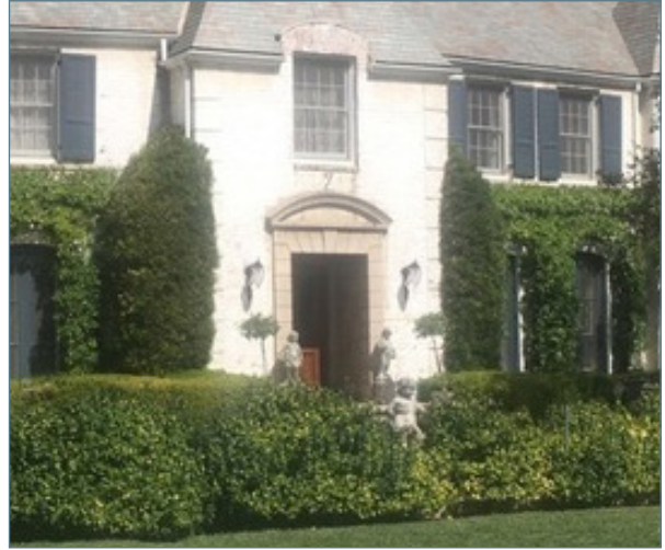
Recessed entrance stoop
