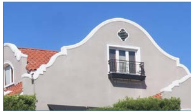
Bell-shaped parapet
