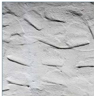
Stucco with different trowel patterns
