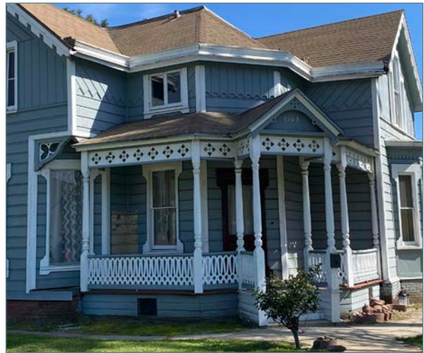
Wraparound porch with wood railing
