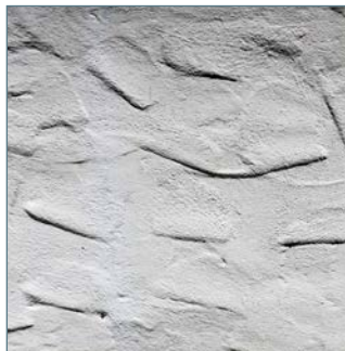
Stucco with different trowel patterns
