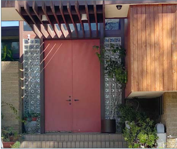
Recessed entrance stoop
