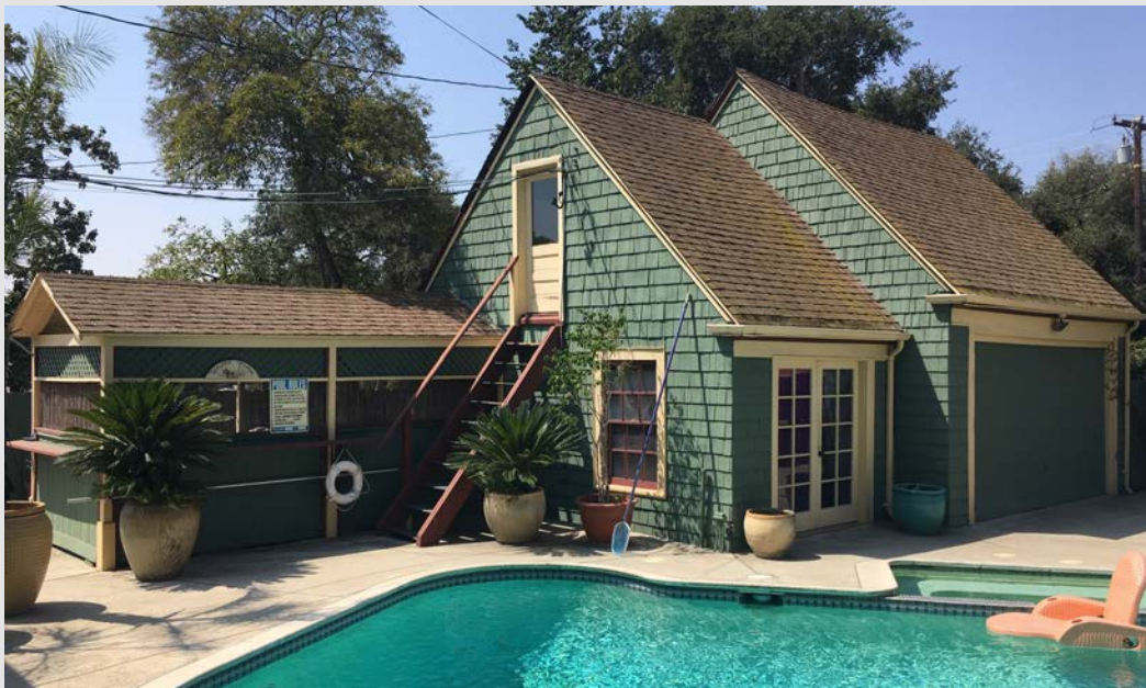
Craftsman carriage house at Victorian Blissner House (210 Orange Grove Ave)
