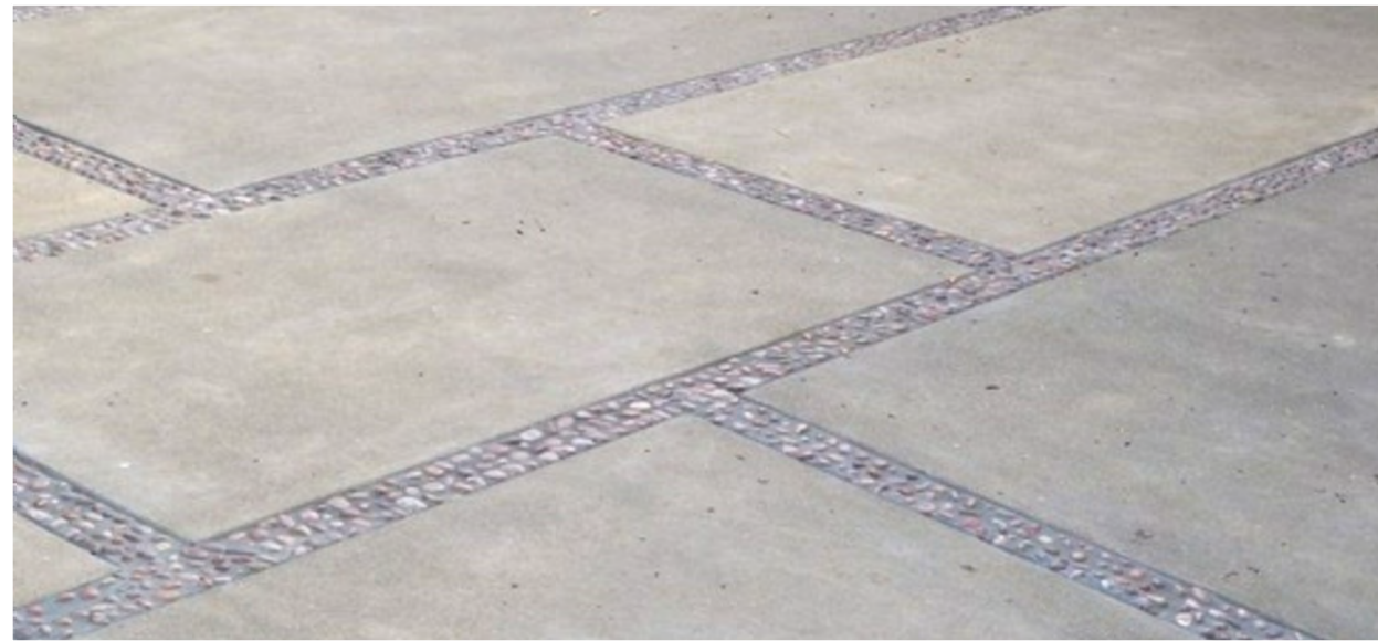
CONCRETE PAVER PATHWAY
