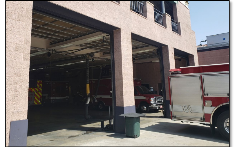
Fire Apparatus Doors
