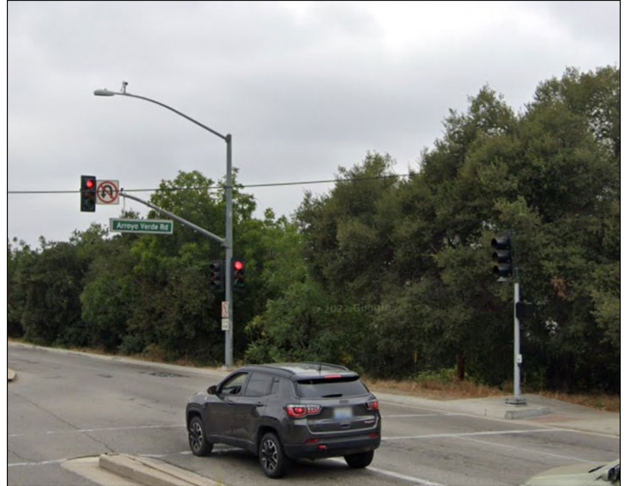
Current Temporary Pole
