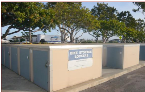
Bicycle Lockers in Marina del Rey
