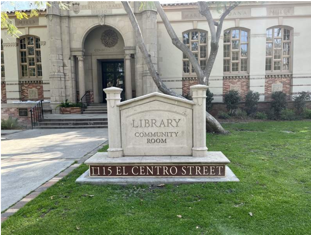
19 - Monument signage is located at the north building entry.
