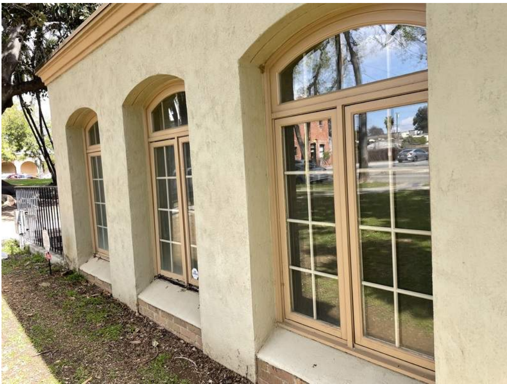
40 - Wooden windows set into exterior cement plaster wall.
