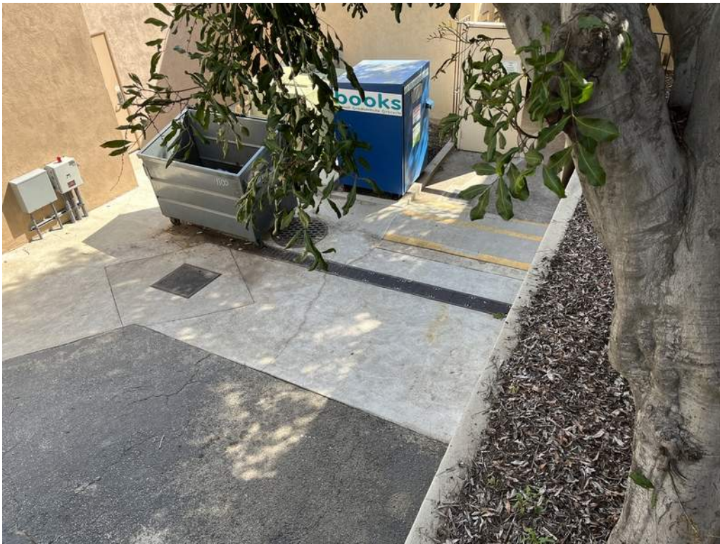
4 - Trench drain at the service yard.
