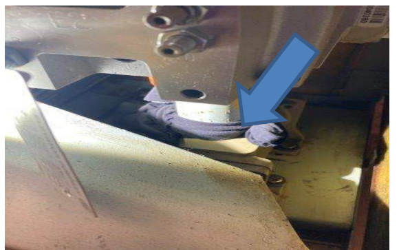
Hydraulic tank hole (top) and Victaulic leak (bottom)
