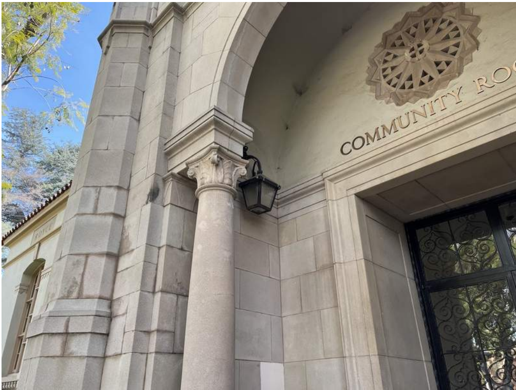
5 - Wall-mounted lantern located at the entrance to the Community Room.
