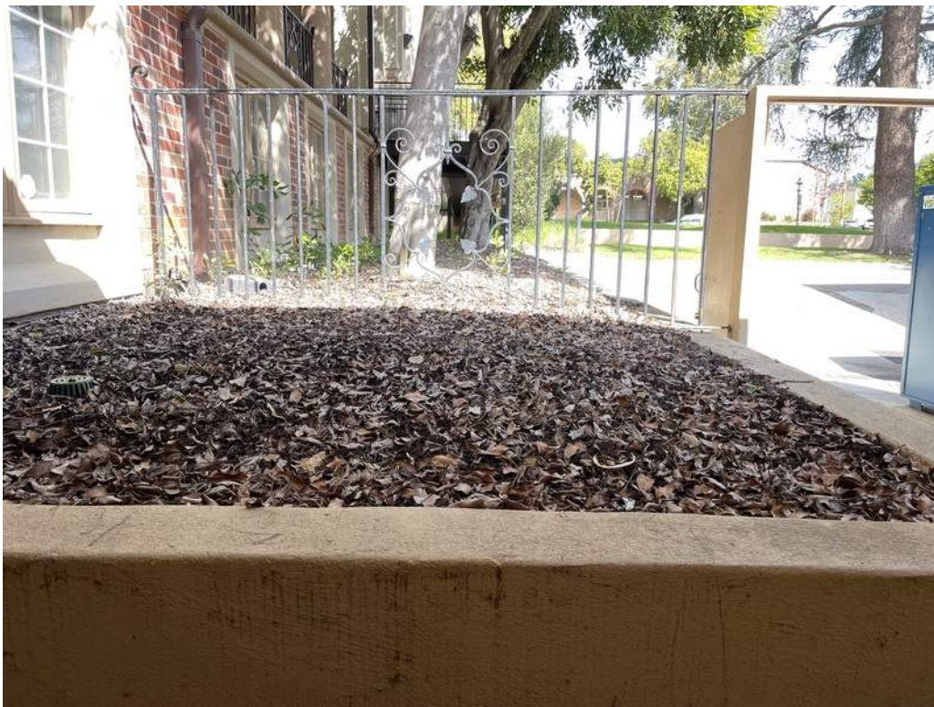
16 - Metal and ornamental fencing at the service yard.
