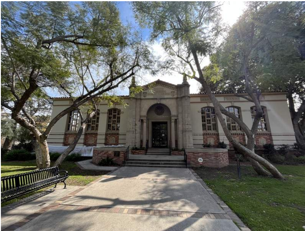
102 - Accessible route without directional signage.
