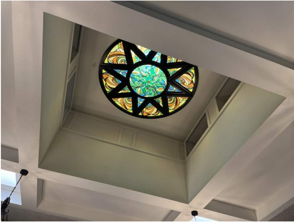
63 - Historic stained glass skylight lens and coffered ceiling at atrium.
