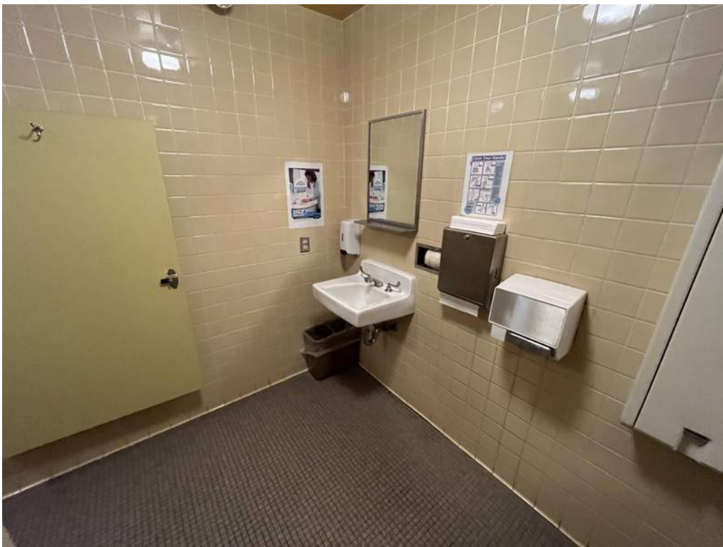
100 - Upper-level women's restroom interior finishes.
