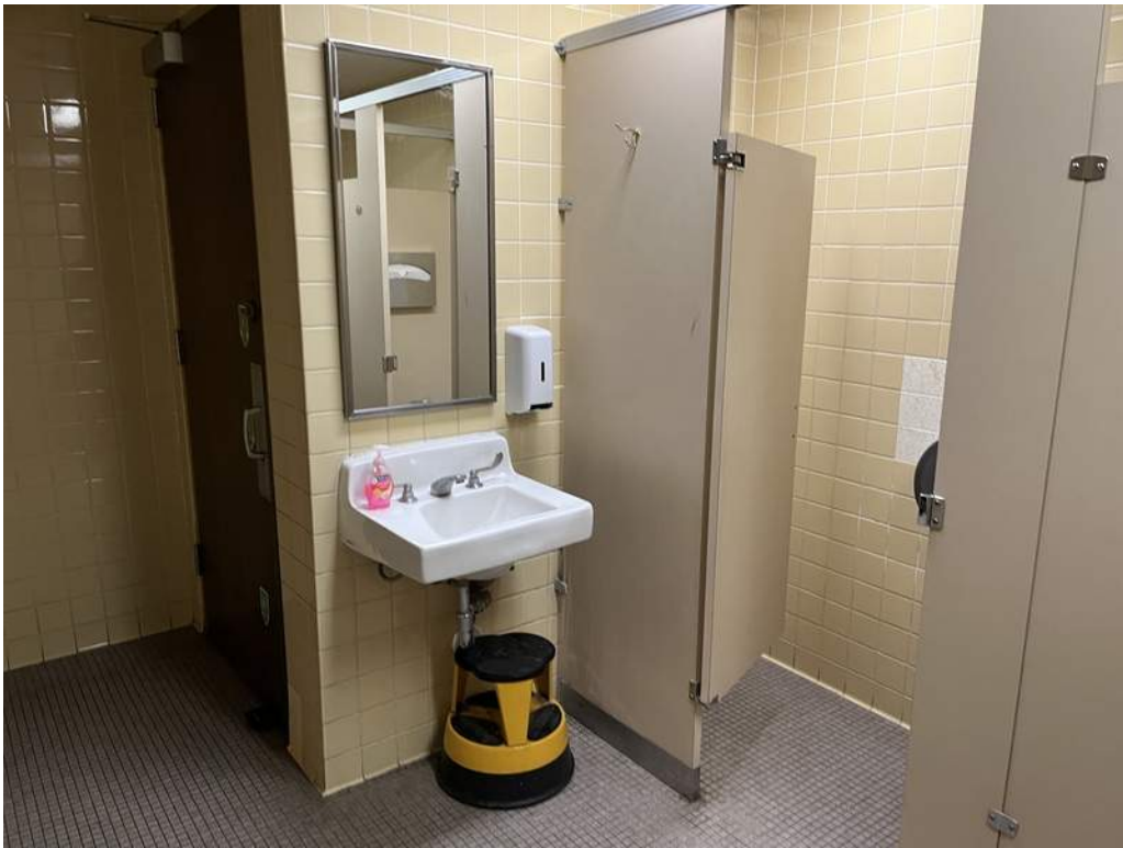
65 - Ground-floor women's restroom interior finishes.
