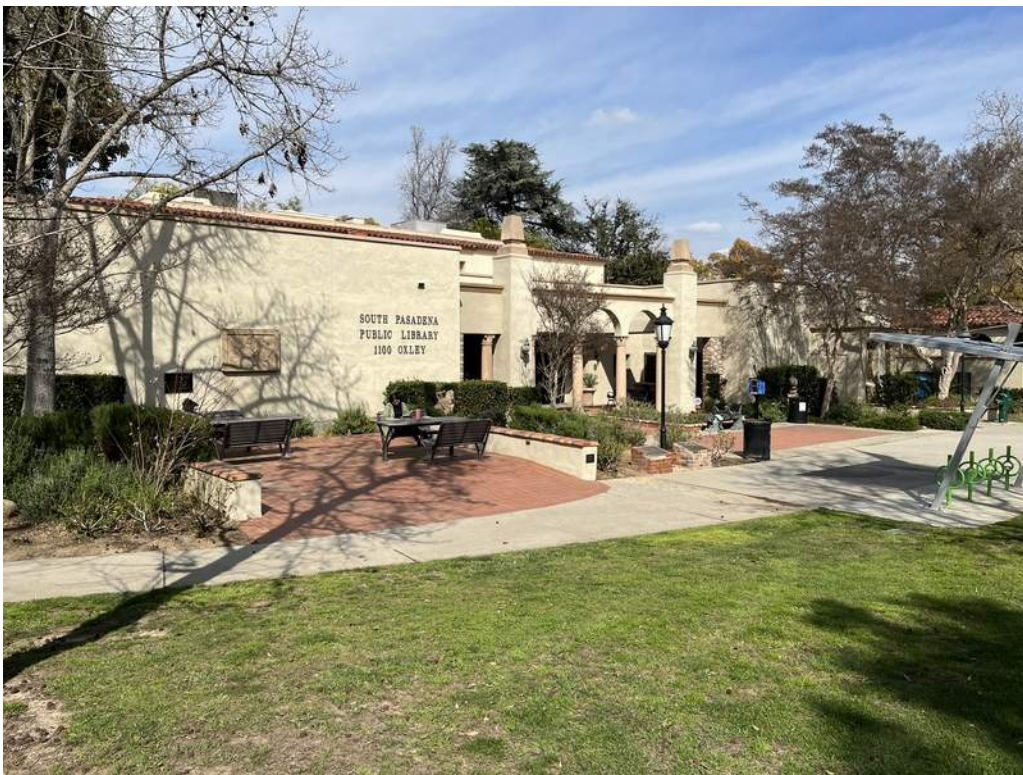
12 - Mowed grass and mature landscaping at the main building entrance plaza.
