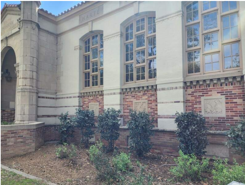
24 - Exterior view of the original 1930 unreinforced masonry.
