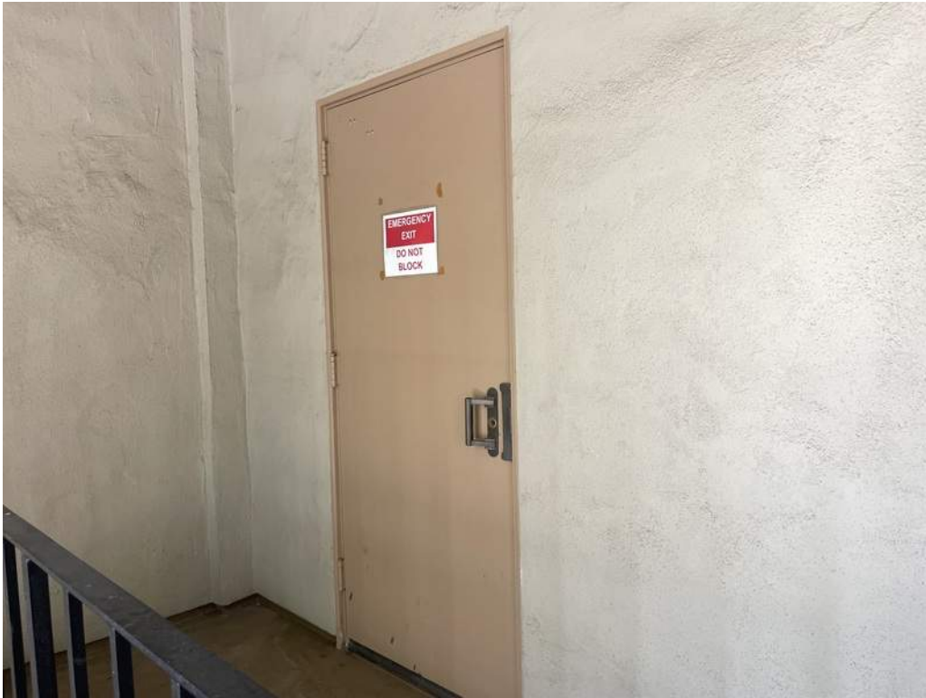
47 - Representative painted hollow metal egress door.
