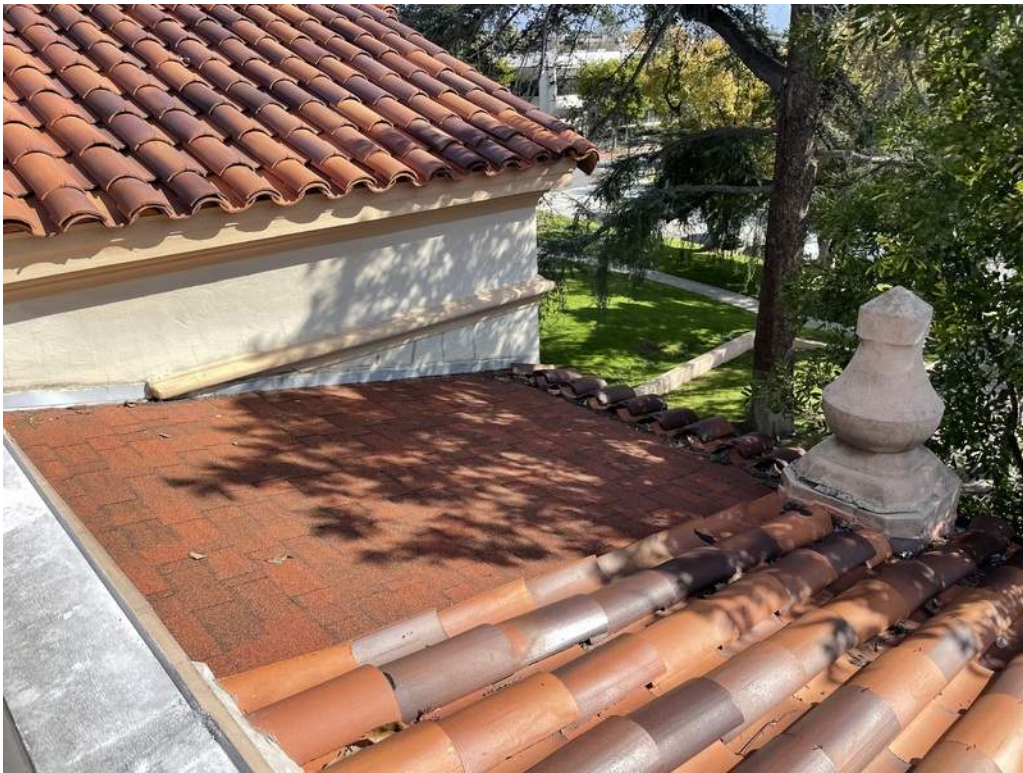
29 - Pitched roof with asphalt singles.
