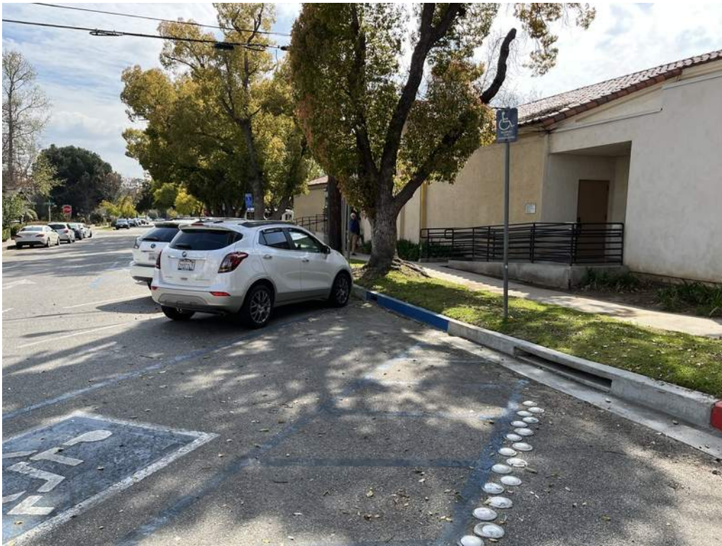
97 - Non-compliant accessible parking spaces without an adjacent curb ramp to the path of travel.
