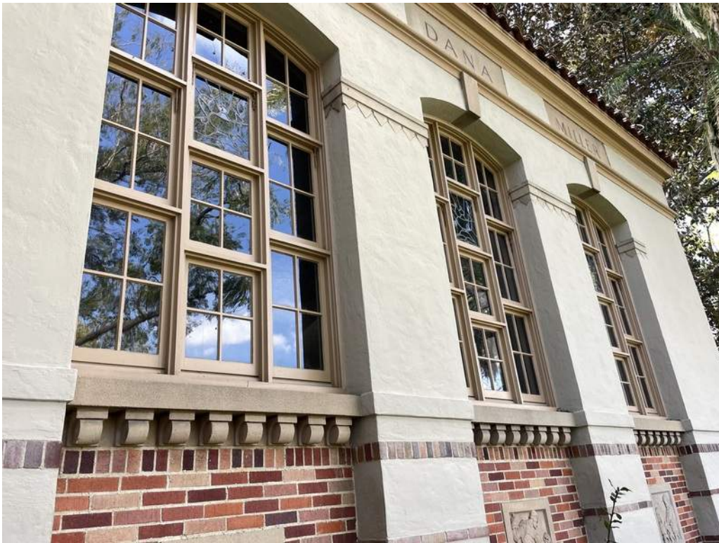
38 - Original wooden windows set into exterior cement plaster wall and accents of brick and stone.
