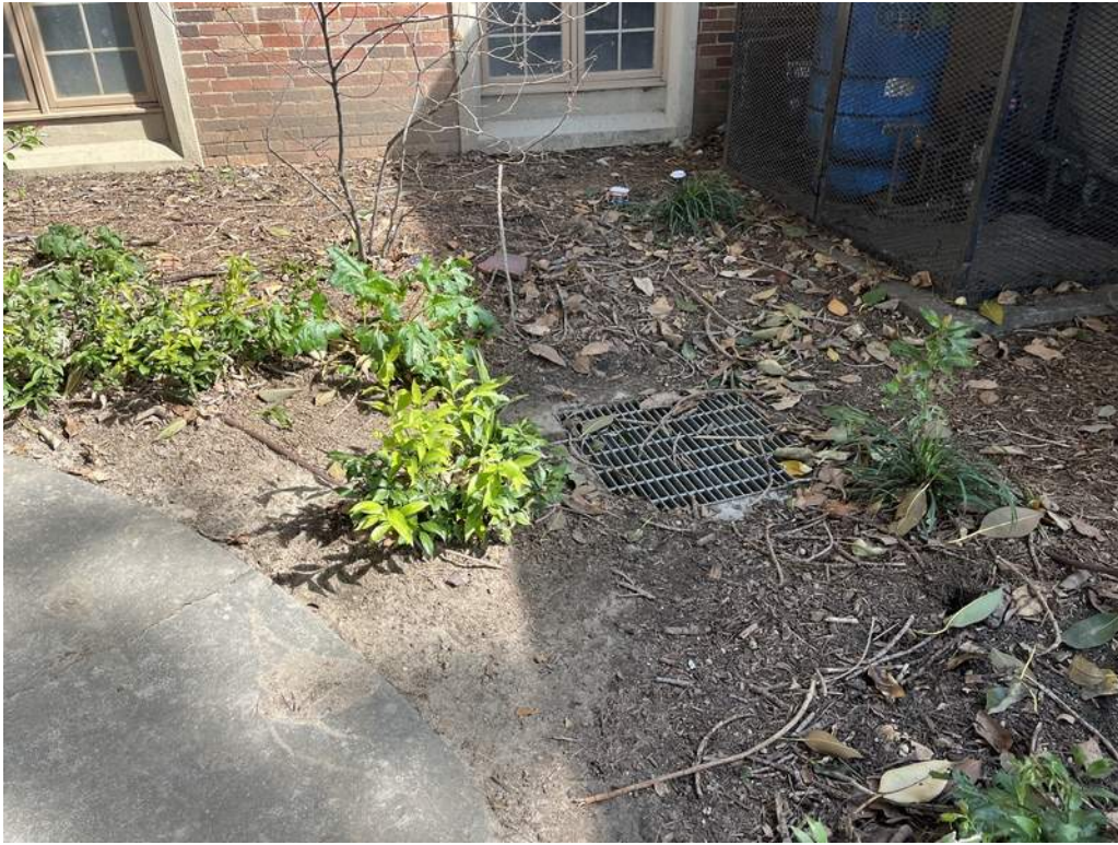
3 - Representative catch basin at the landscaped areas.
