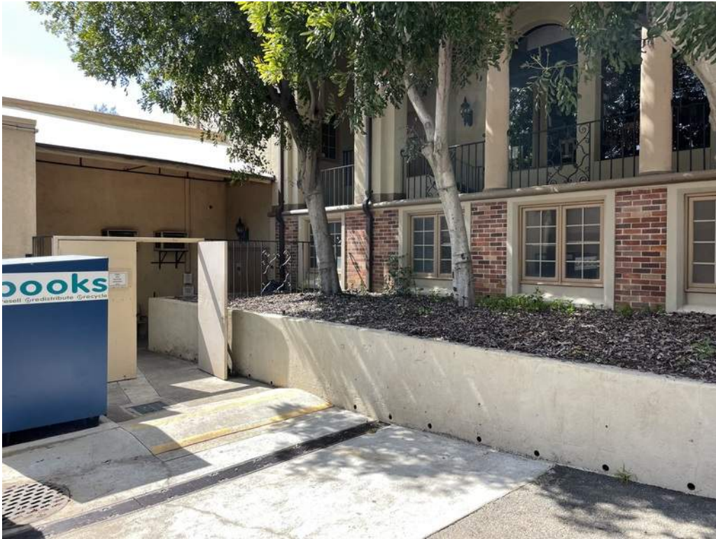
15 - Retaining planter on the east side of the building.
