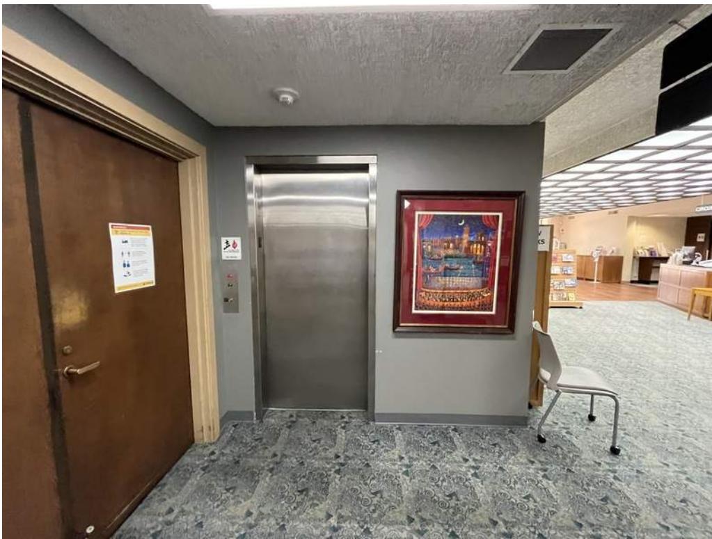
58 - Ground-floor elevator lobby interior finishes.
