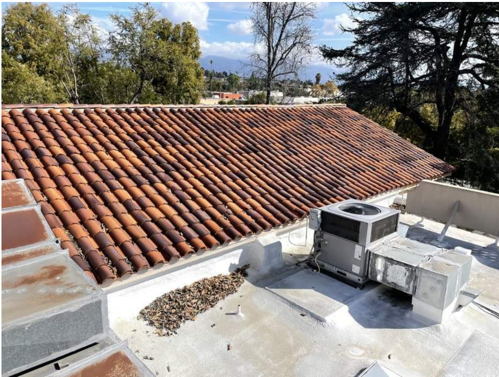
28 - Pitched roof with tapered barrel single-piece clay tiles.
