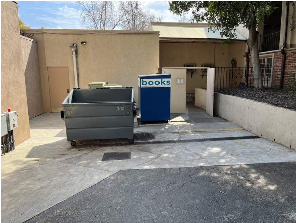
8 - Overview of the rear service yard.
