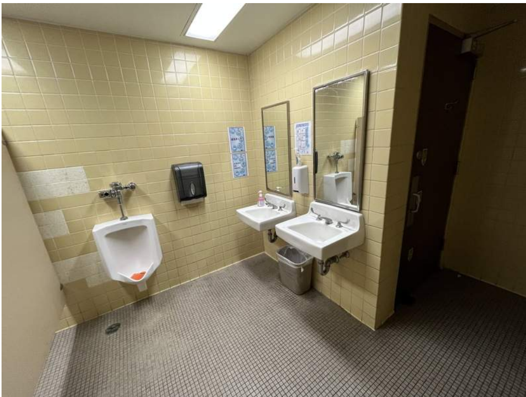
98 - Ground-floor men's restroom interior finishes.
