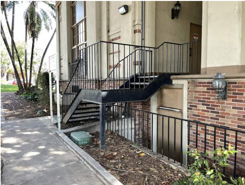
49 - West balcony steel-framed egress stairs and handrails with painted finish.
