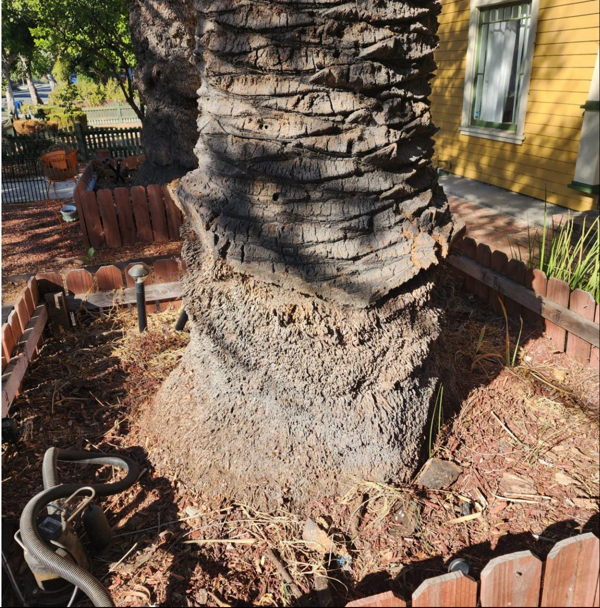
Palm Tree #2 (Notice the soil grade has been raised around the base of the tree)
